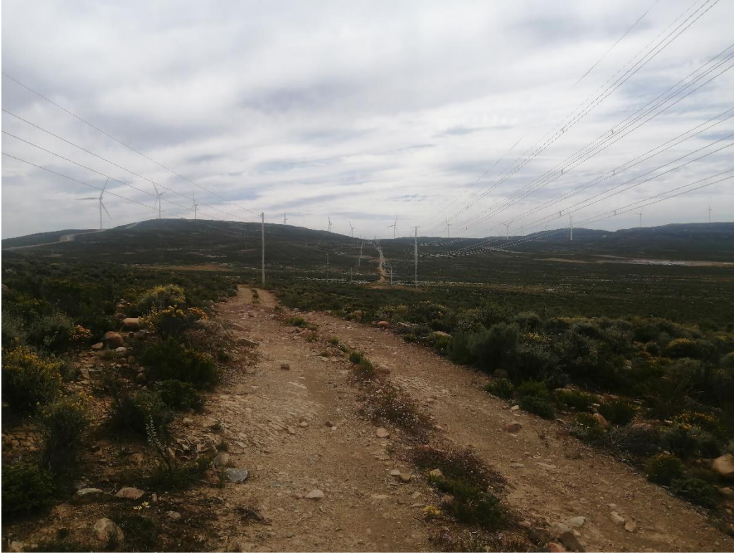
Figure 5: View of access road used along the 132kV powerline.
