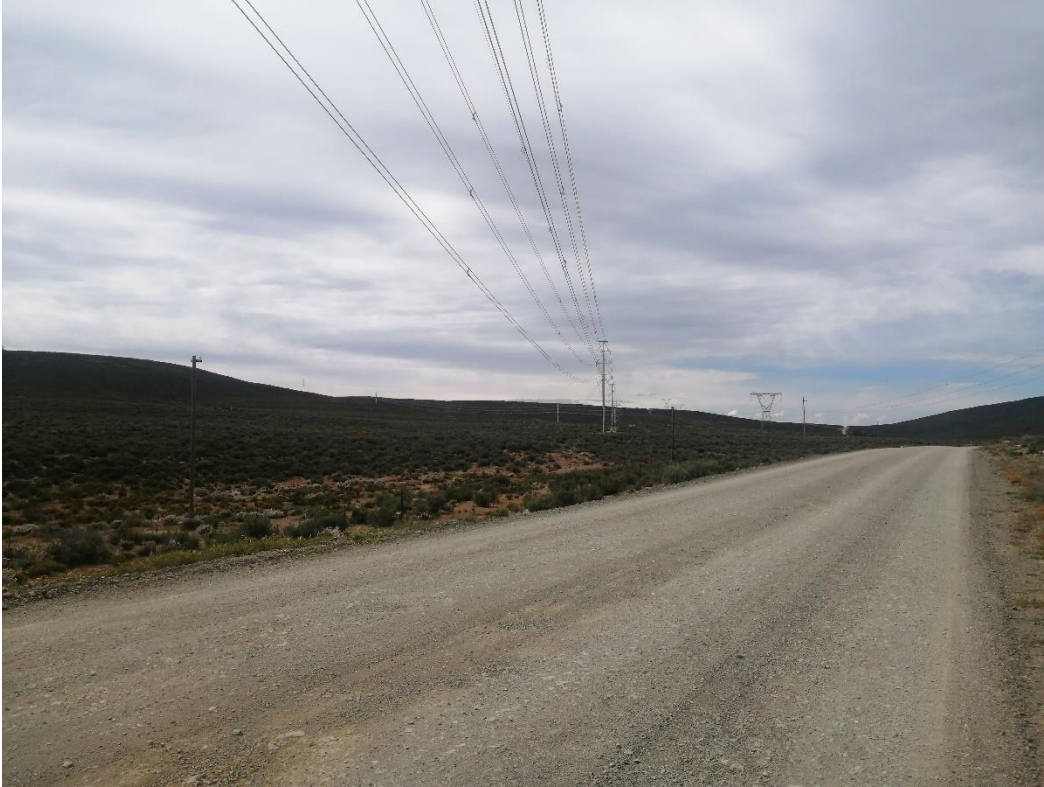
Figure 7: View of the 132kV overhead powerline road crossing.
