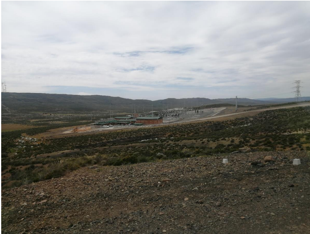
Figure 3: View of the Karusa substation.
