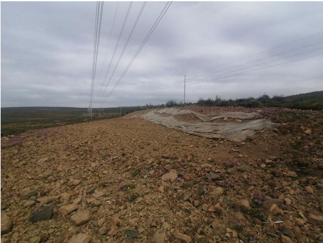
Figure 6: View of an area previously sloped to achieve conductor ground clearance.
