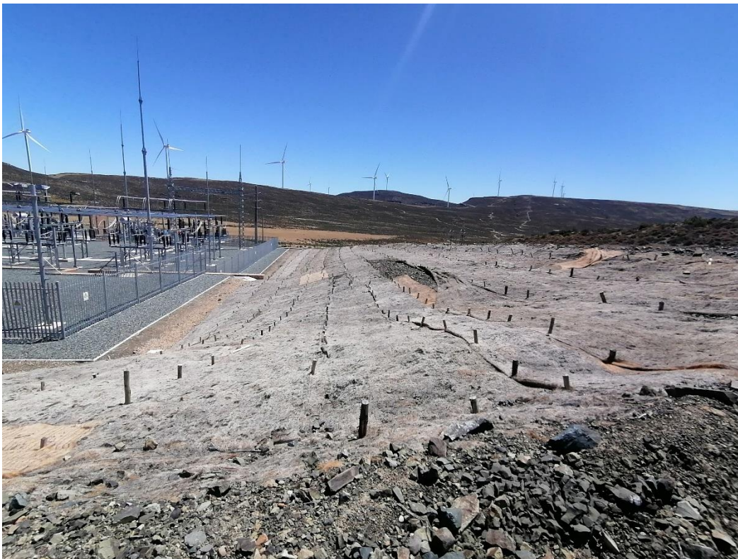
Figure 4: View of reinstated slopes adjacent to the Karusa Substation.
