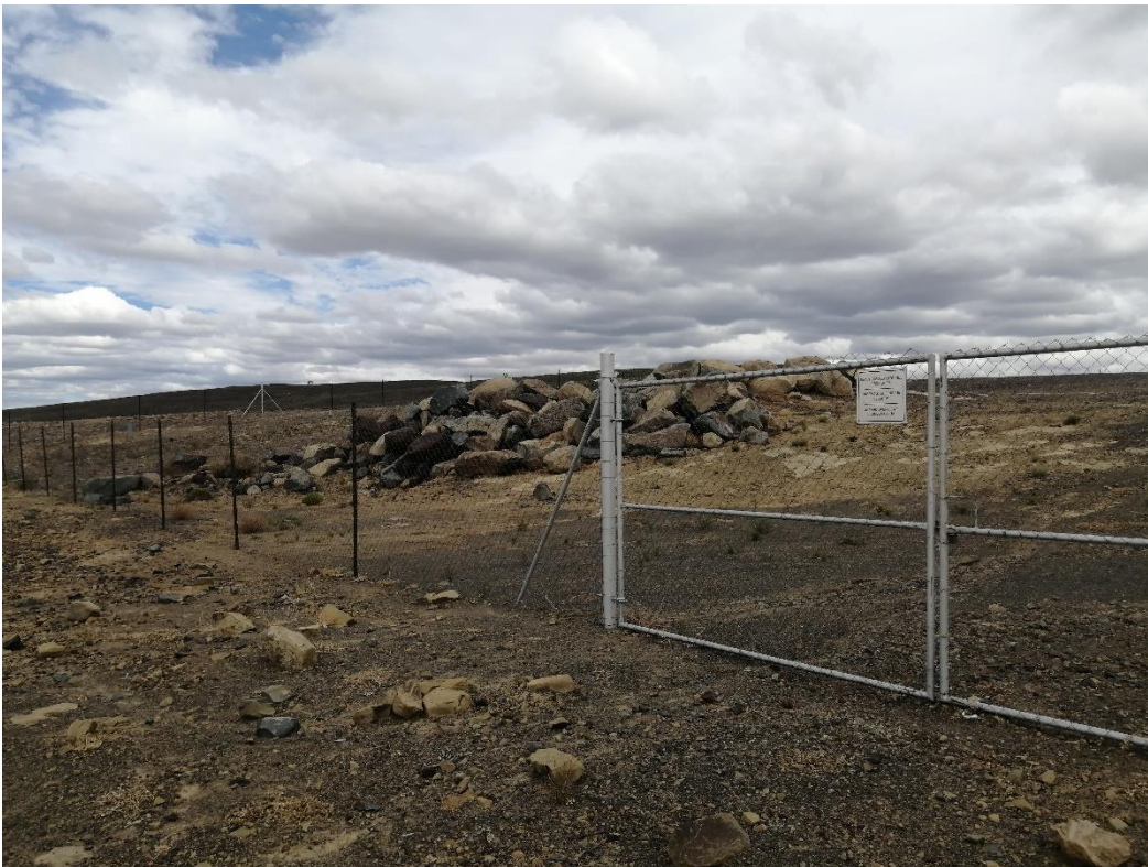
Figure 12: View of the crushing area along road 6.
