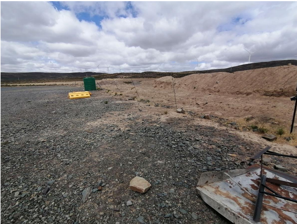
Figure 8: View of topsoil windrowed along the western boundary of the main camp.
