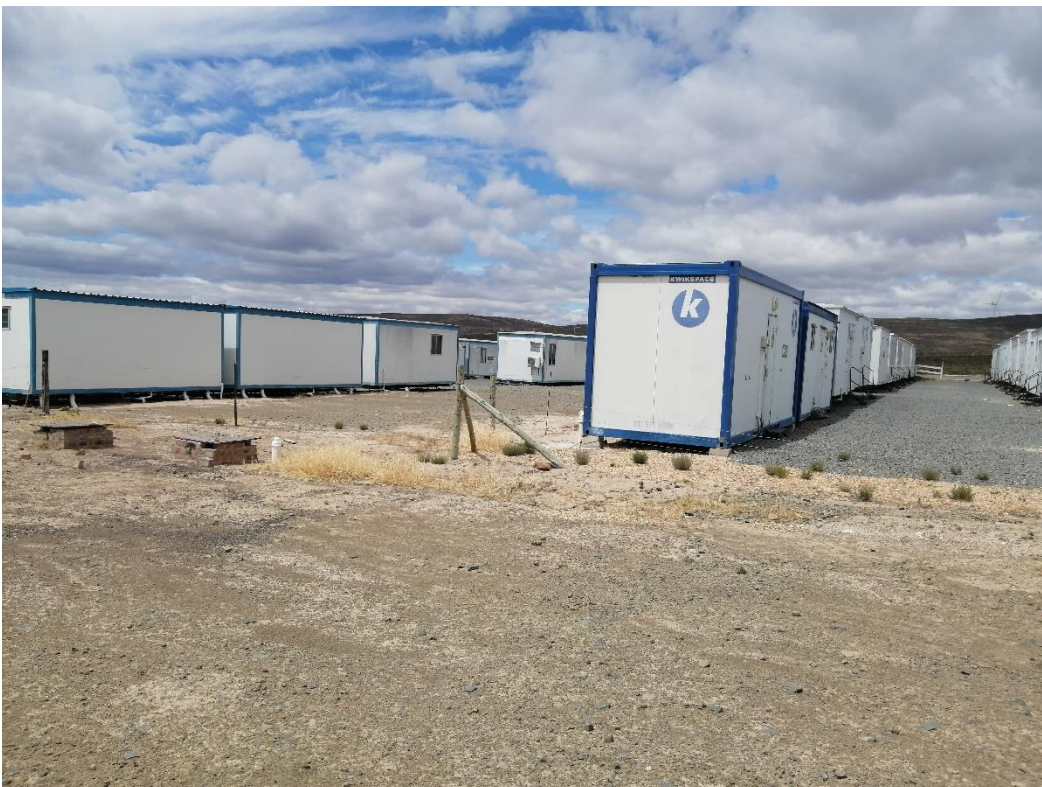
Figure 6: View of office containers remaining at the main camp.
