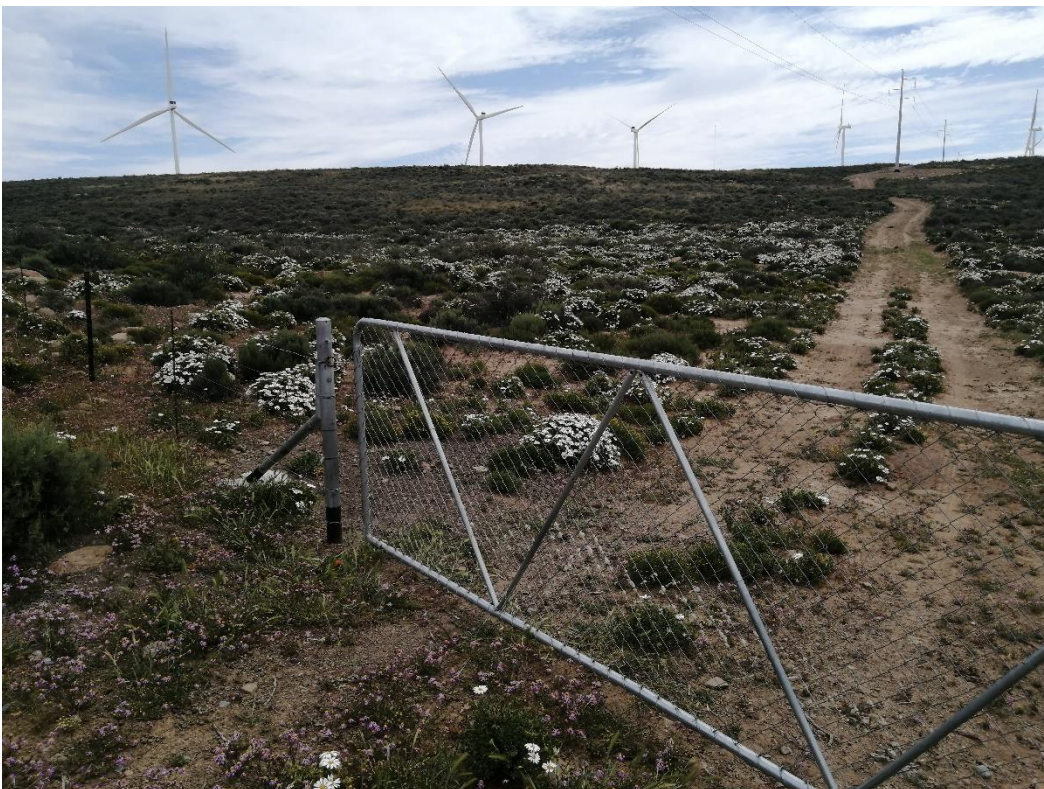
Figure 6: Most gates were noted either closed or locked during the audit inspection.
