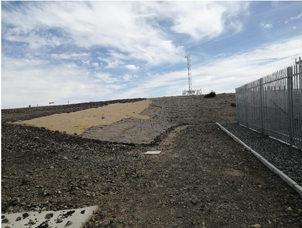
Figure 3: View of slope stabilisation efforts outside the Soetwater substation.
