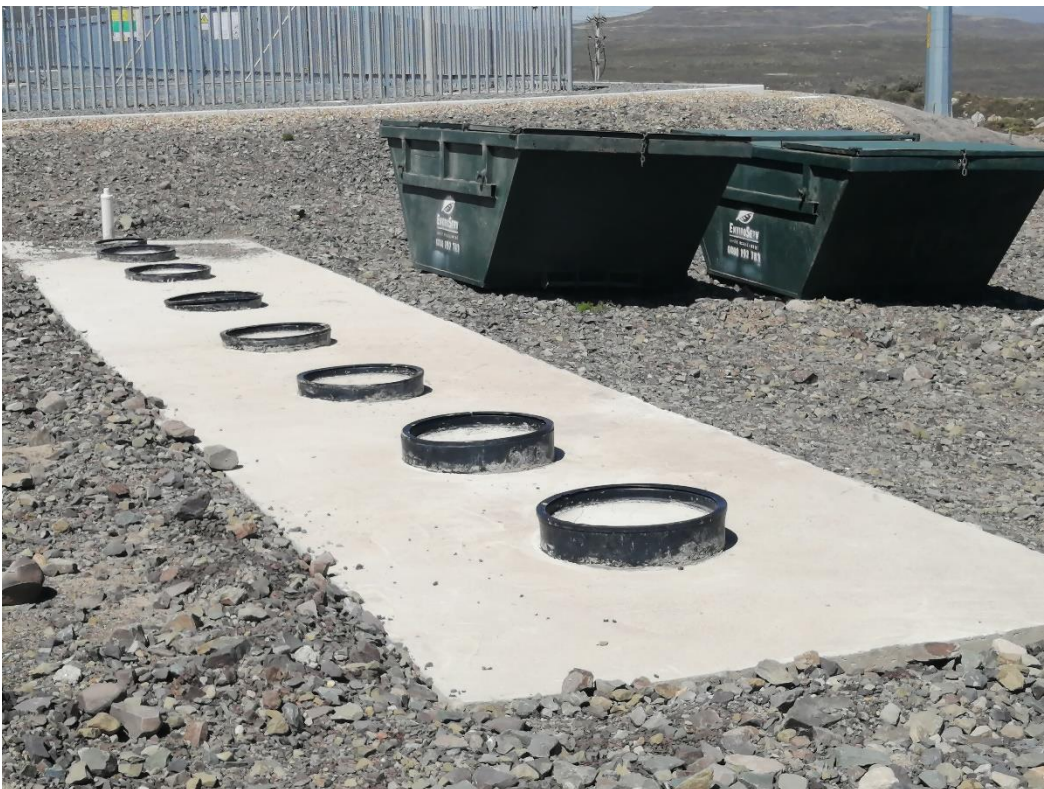
Figure 6: View of waste skips used at the Soetwater Substation.
