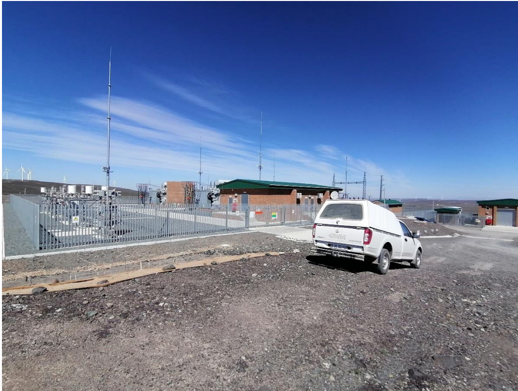
Figure 3: View of the Soetwater substation.
