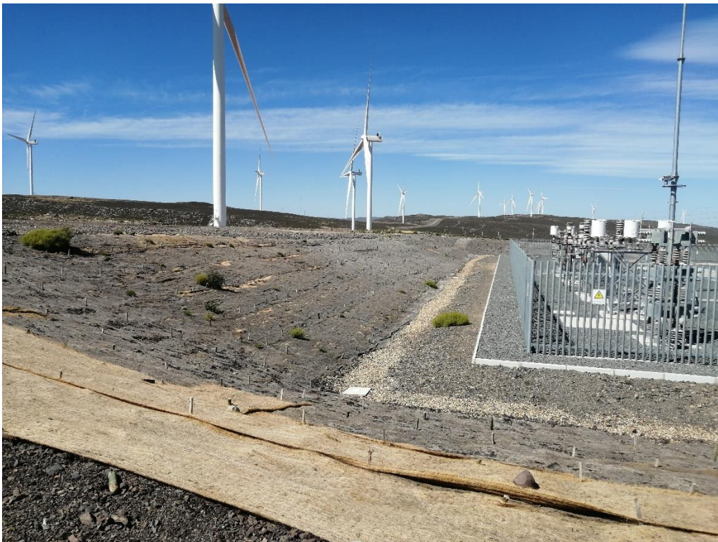
Figure 4: View of reinstated slopes adjacent to the Soetwater Substation.
