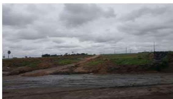
Figure 16: Main haul and access road.
