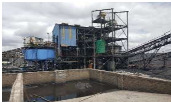
Figure 5: Processing/ beneficiation plant- westside plant, ptn 7.
