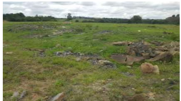
Figure 20: Inadequately rehabilitated western opencast.
