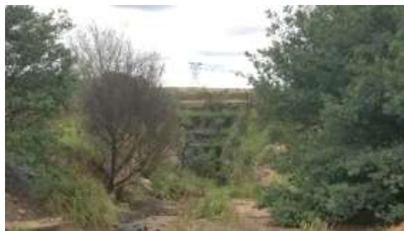
Figure 3: South eastern decline shaft.
