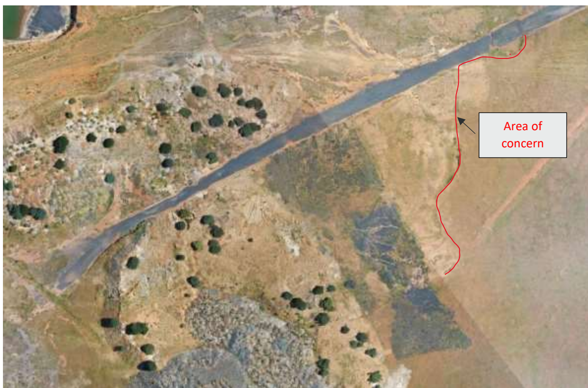
Figure 64: Possible settlement of backfilled areas.
