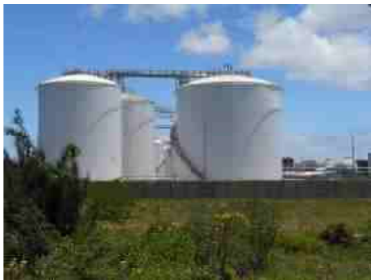
Figure 1: Photo of the IVS Storage Facility in the Port of Richards Bay South Dunes Precinct.
