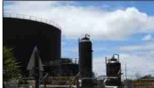
Figure 8: Photo of the JBS Storage Facility
