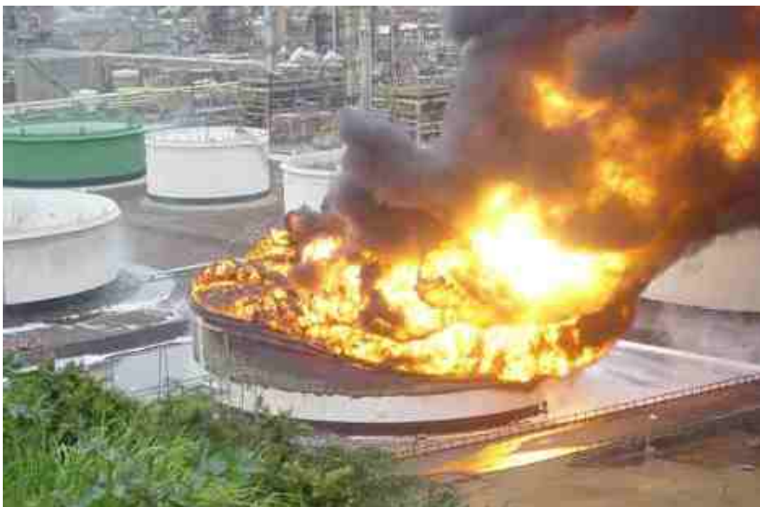
Figure 7: Tank-top fire at the Engen refinery caused by lightning
