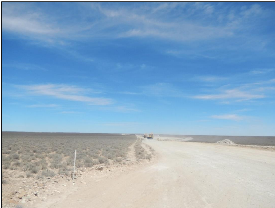
Figure 19: View of the construction activities associated with the proposed Khobab Wind Farm.
