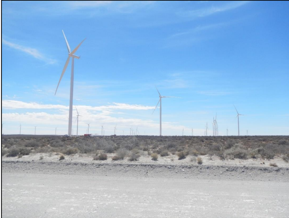
Figure 16: Wind turbines at the Loeriesfontein Wind Farm
