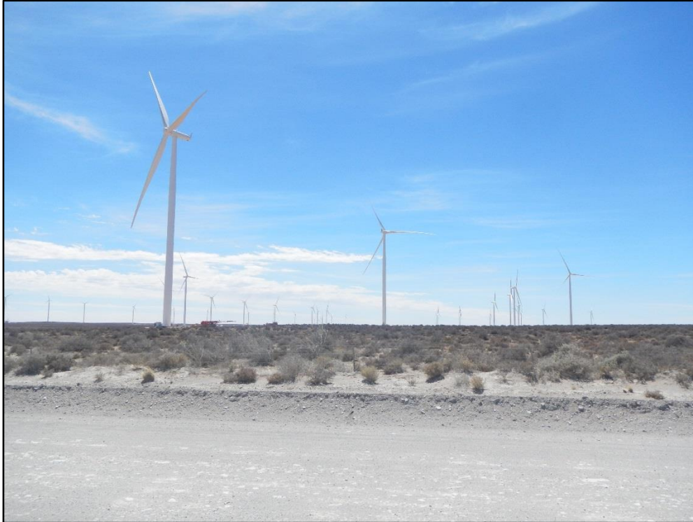
Figure 16: Wind turbines at the Loeriesfontein Wind Farm.
