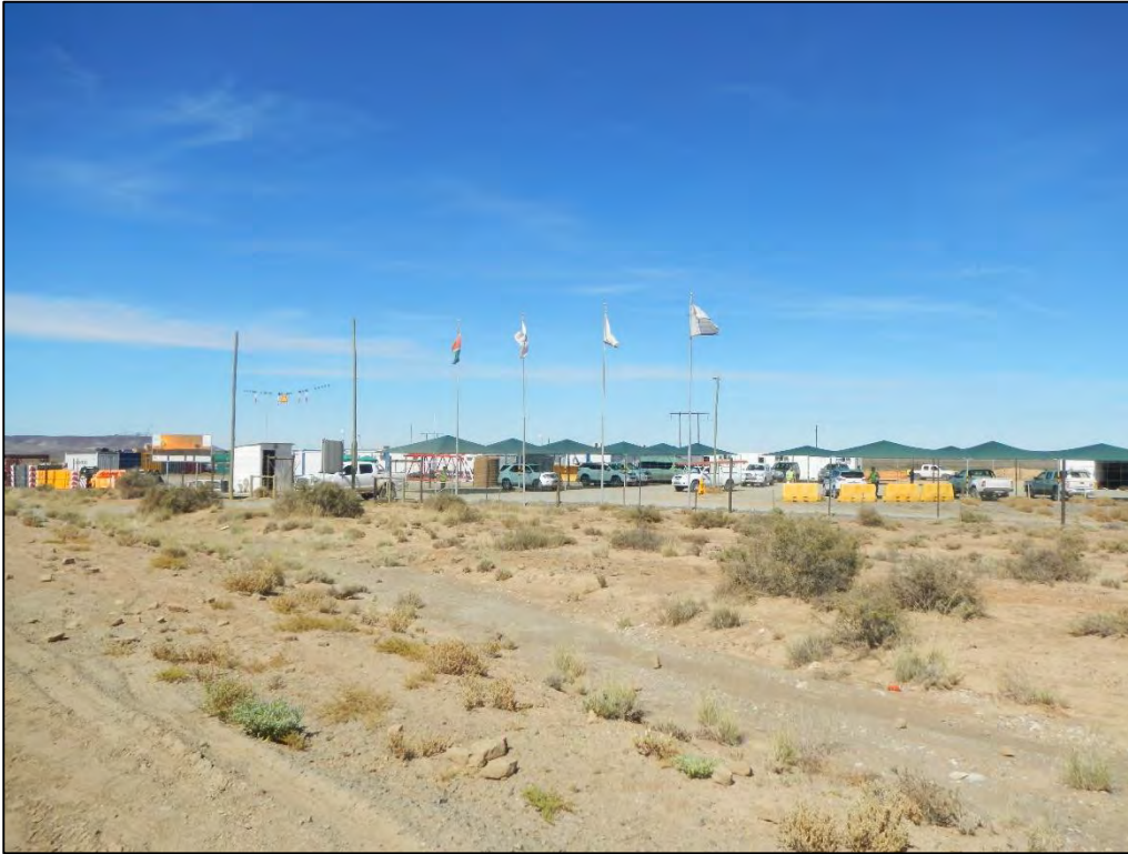
Figure 108: View of the Khobab Wind Farm construction camp area which is situated at the Helios Substation. This construction camp is however situated well outside of the visual assessment zone
