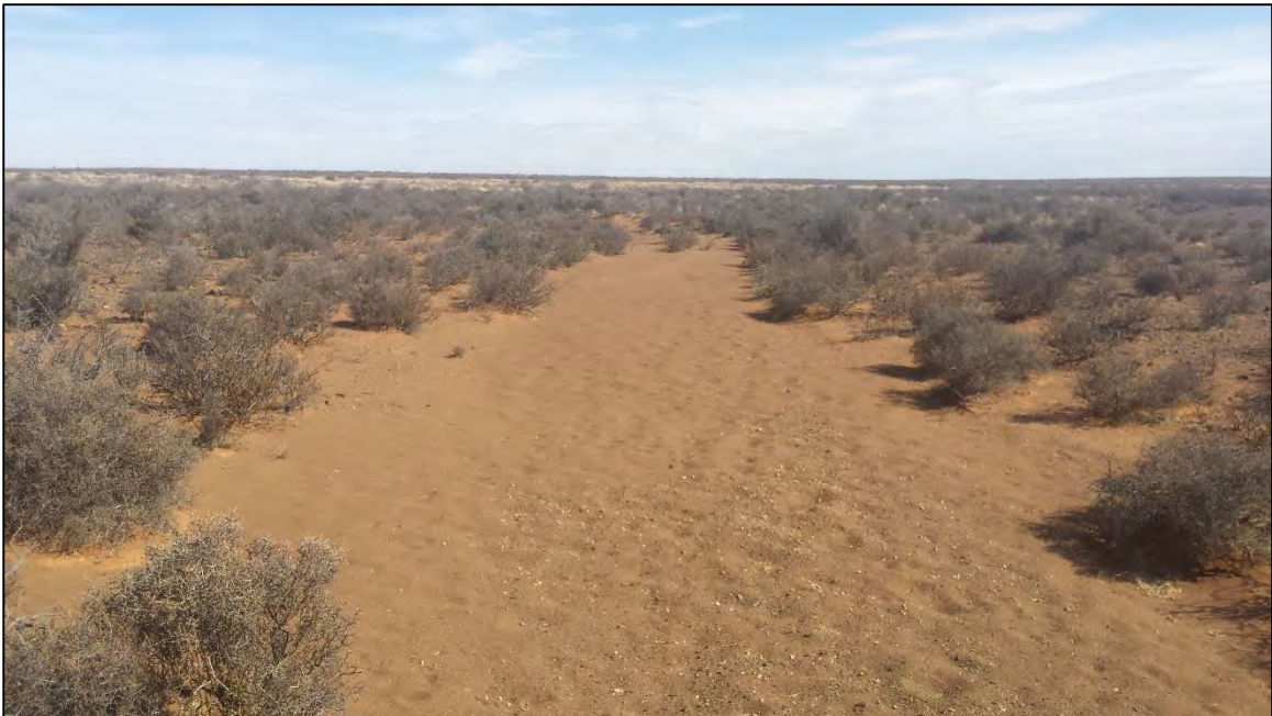
Figure 83: Example of Deposited Sand within a Drainage Line
