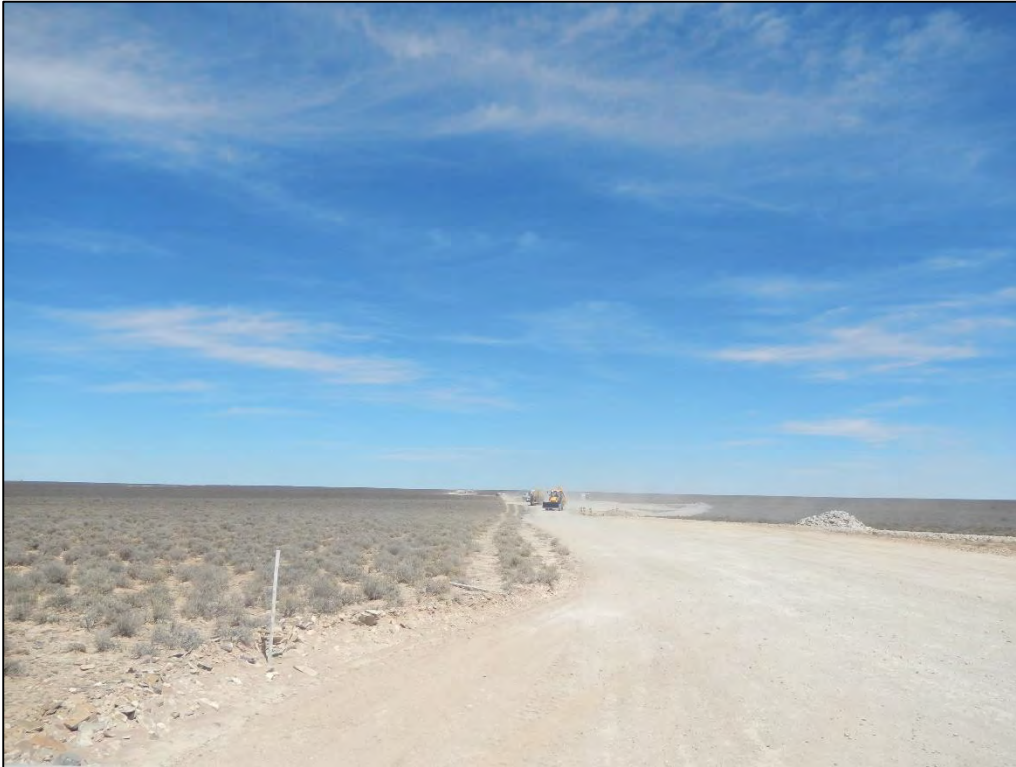
Figure 109: View of the construction activities associated with the proposed Khobab Wind Farm. During the time of the in-field investigation it was noted that this wind farm was still in the early stages of construction and no turbines had thus been erected.
