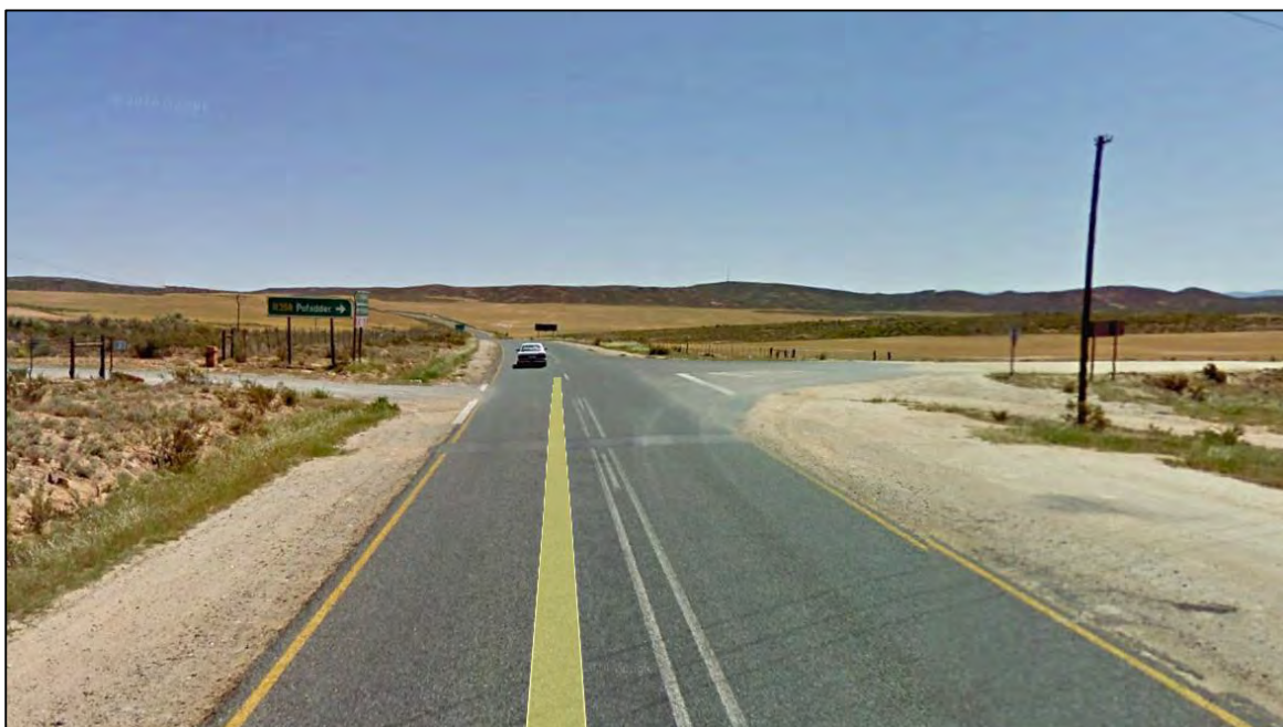
Figure 141: N7 / R358 Intersection
