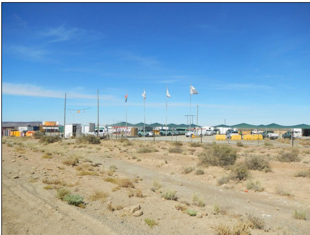
Figure 97: View of the Khobab Wind Farm construction camp area which is situated at the Helios Substation. This construction camp is however situated well outside of the visual assessment zone
