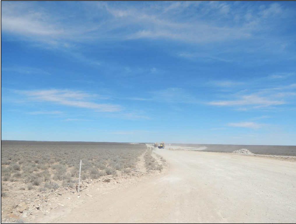
Figure 98: View of the construction activities associated with the proposed Khobab Wind Farm. During the time of the in-field investigation it was noted that this wind farm was still in the early stages of construction and no turbines had thus been erected.
