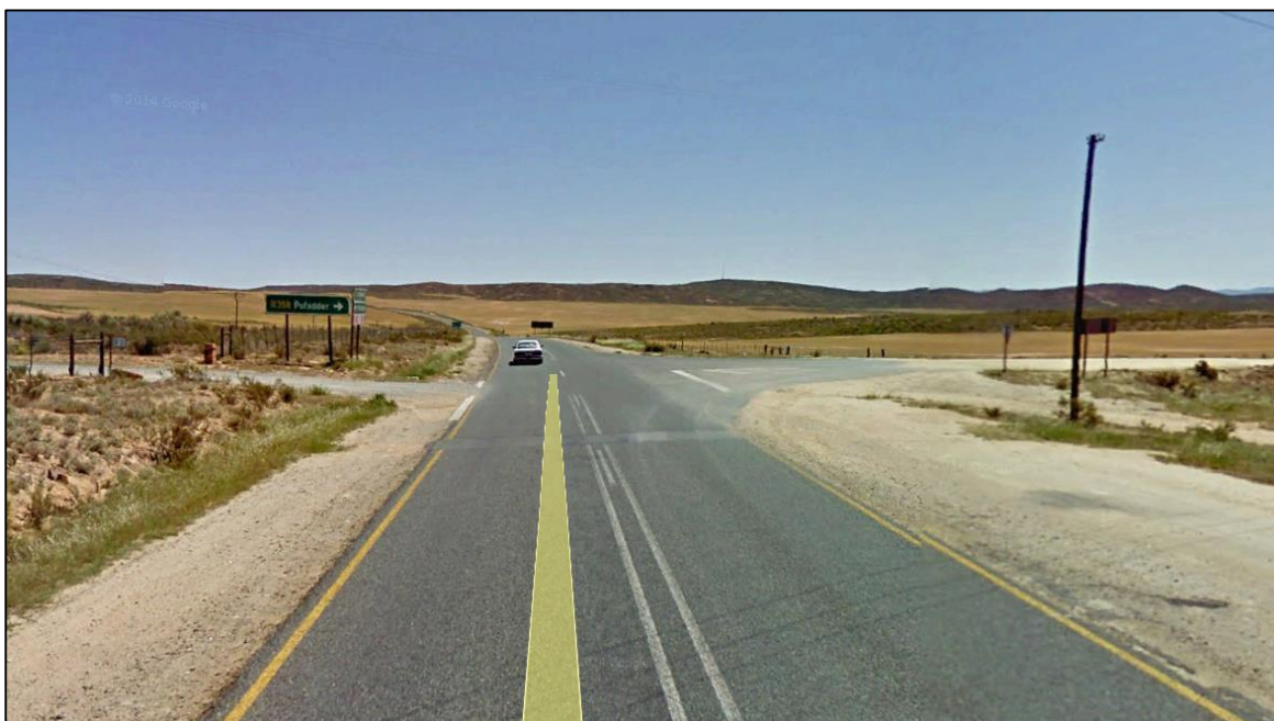
Figure 112: N7 / R358 Intersection
