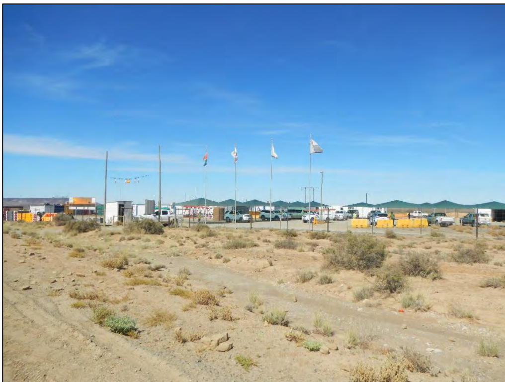
Figure 102: View of the Khobab Wind Farm construction camp area which is situated at the Helios Substation. This construction camp is however situated well outside of the visual assessment zone
