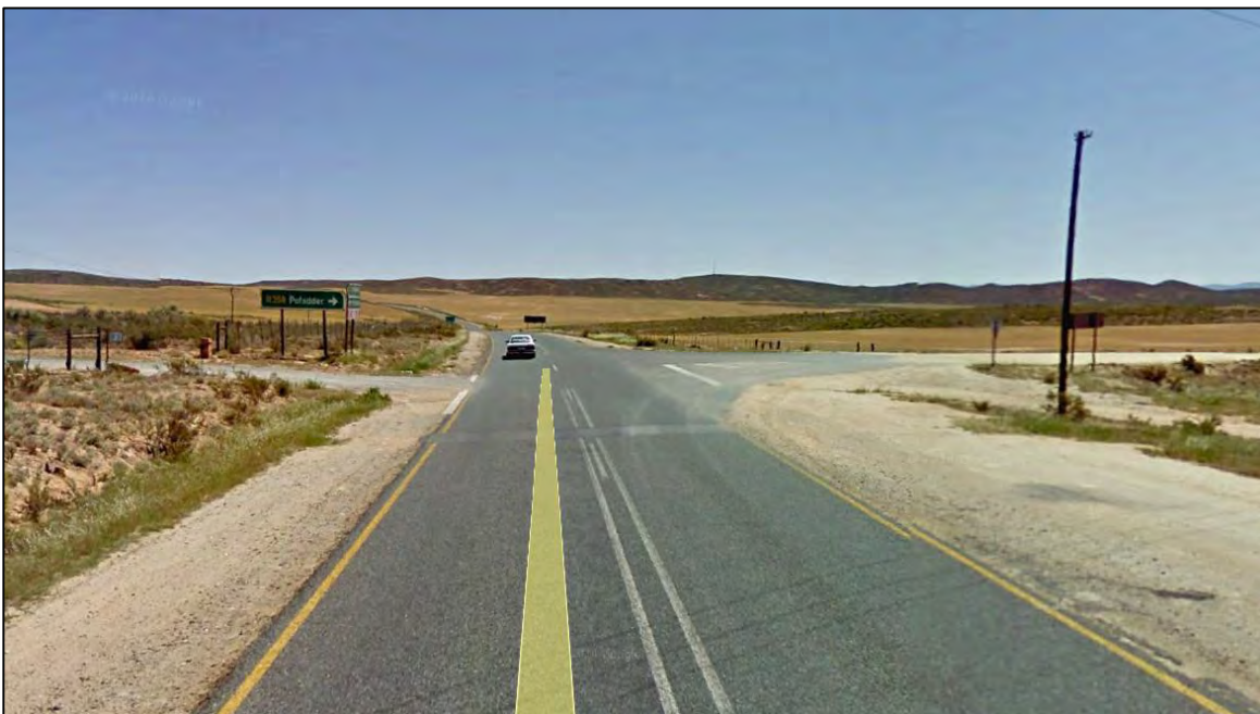
Figure 141: N7 / R358 Intersection
