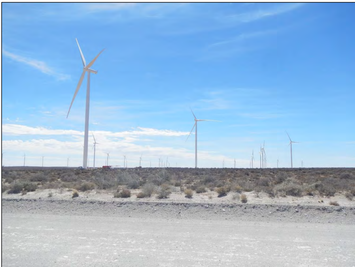
Figure 32: View of the Loeriesfontein Wind Farm which has been constructed approximately 23km to the east of the proposed Hartebeest Leegte Wind Farm application site. This wind farm is however located
