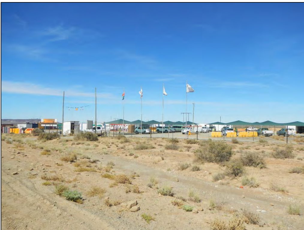
Figure 97: View of the Khobab Wind Farm construction camp area which is situated at the Helios Substation. This construction camp is however situated well outside of the visual assessment zone
