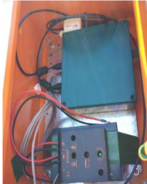
Figure 48: SM2BAT+ detector and supporting hardware
