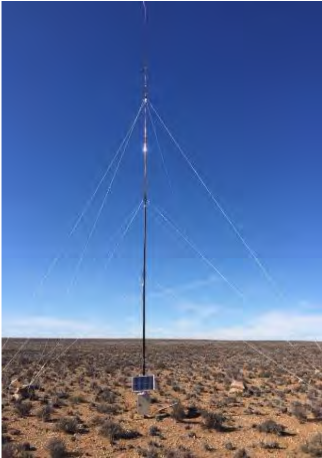
Figure 47: Short mast monitoring system
