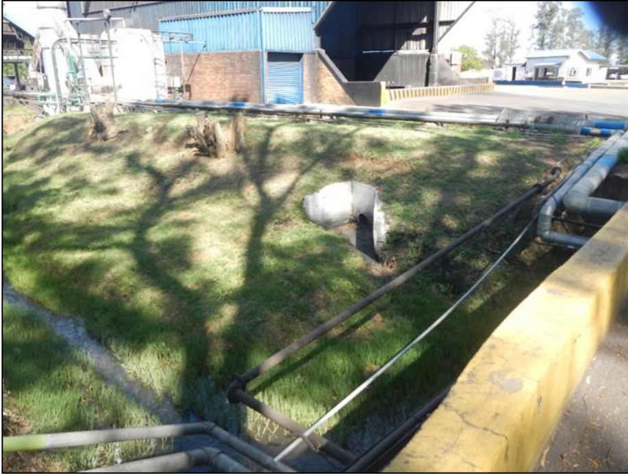
Figure 7: Storm water outlets directing storm water run-off into the Kok's River
