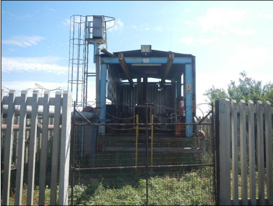
Figure 2: Pump Station found within close proximity to the Kliprivier. Used to draw water from the river in case of fire outbreaks only.
