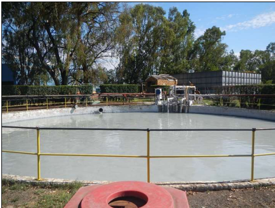
Figure 5: Holding dam used to store the treated effluent on site before it is discharged into the municipal system
