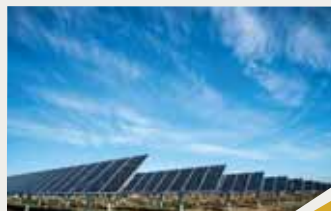
New 132kV Impala Switching Station and 132/11kV, 1x 80MVA Sishen Solar Facility Substation
