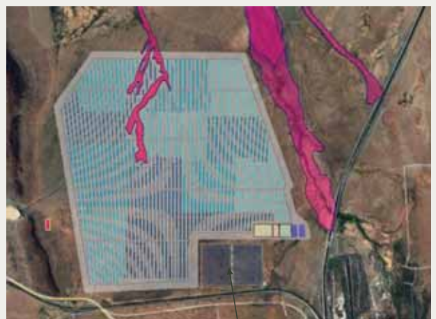
De Aar 10MW solar plant
