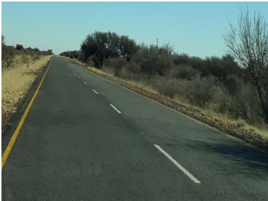
Photograph 3.1: Road condition R31
