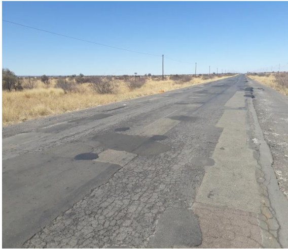
Photograph 3.3: Patching along the route
