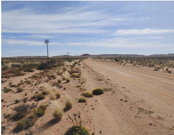
Photo 3: SSD to the North along the R358 from the Access 3 West (>500m)
