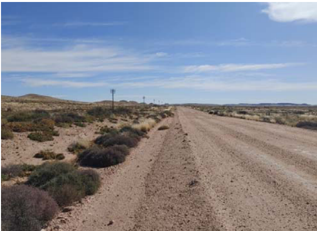
Photo 5: SSD to the North along the R358 from Access 4 (>500m)
