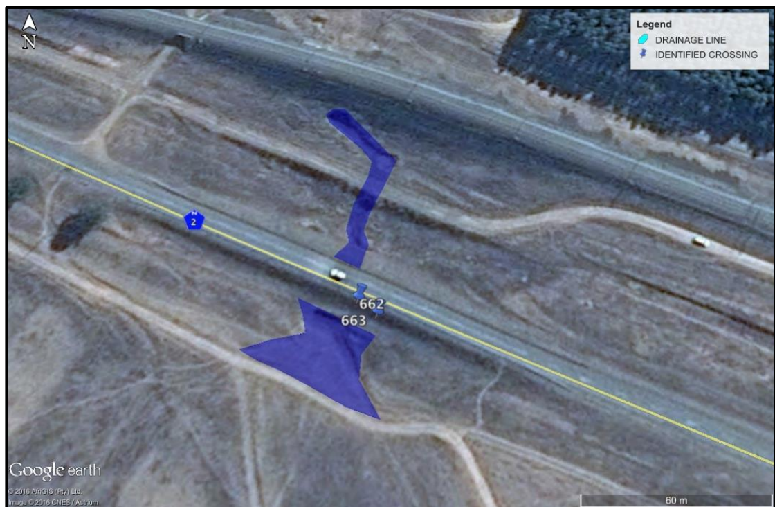
Figure 19: 662 & 663 - Drainage lines and stormwater culverts
