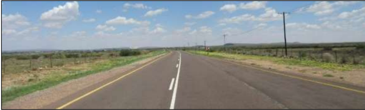
Photograph 3.1: N14, looking west (towards Keimoes) from the entrance to Dyason’s Klip farm
