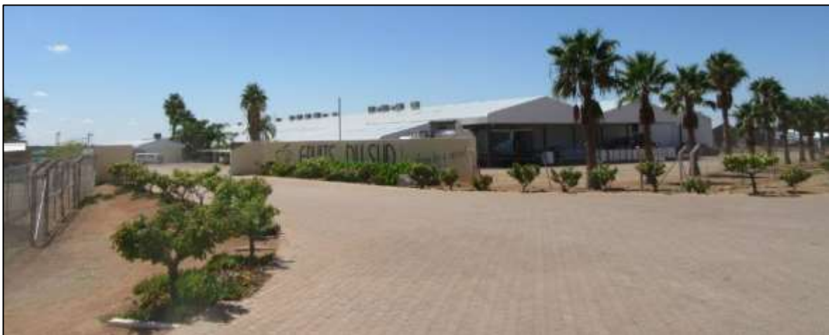
Photograph 3.6: Fruits de Sud's raisin processing facility near the N14-Kanoneiland Road intersection
