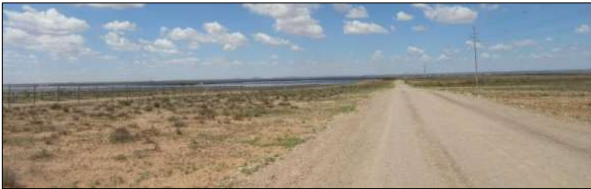
Photograph 3.13: Daysonklip 1 SEF (left) and 132 kV Dyasonsklip line seen from south of the Dyasonsklip SEF substation
