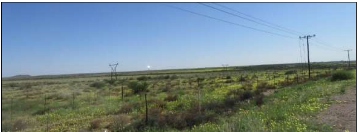
Photograph 3.10: Existing Eskom and Telkom lines located 200 m to the north of the N14
