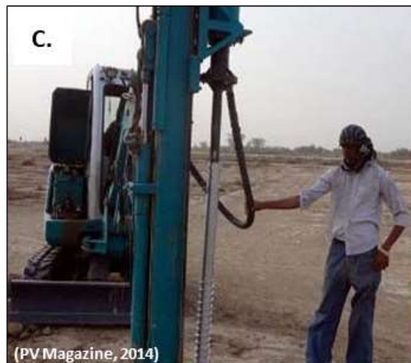
Figure 7: Mounting Structures. A) Cast Concrete Foundation. B) Driven/ Rammed Steel Pile. C) Ground / Earth Screw.
