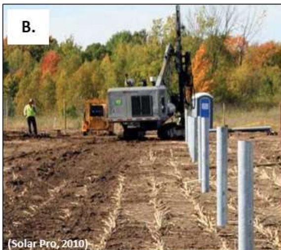
Figure 7: Mounting Structures. A) Cast Concrete Foundation. B) Driven/ Rammed Steel Pile. C) Ground / Earth Screw.
