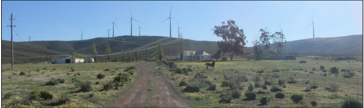
Photograph 3.14: Farmstead and outbuildings on Bon Espirange seen from entrance road. Note the turbines (Roggeveld WEF) and overhead lines feeding into on site Roggeveld WEF substation. The impact is contained to the west and south of the farmstead
