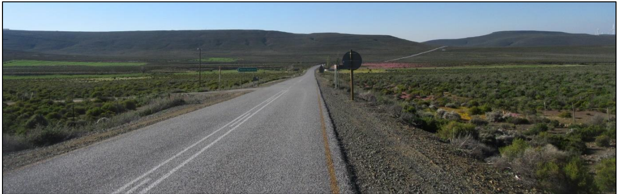
Photograph 3.2: R354 looking north from near entrance to Swartland and Bon Espirange farms
