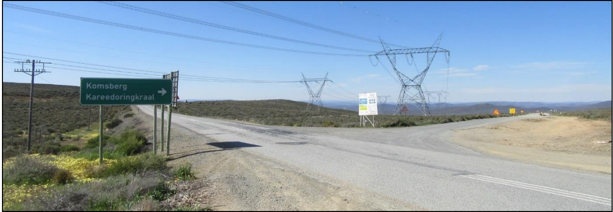
Photograph 3.1: R354-Komsberg road intersection and 756 kV and 400 kV lines viewed from the south.
