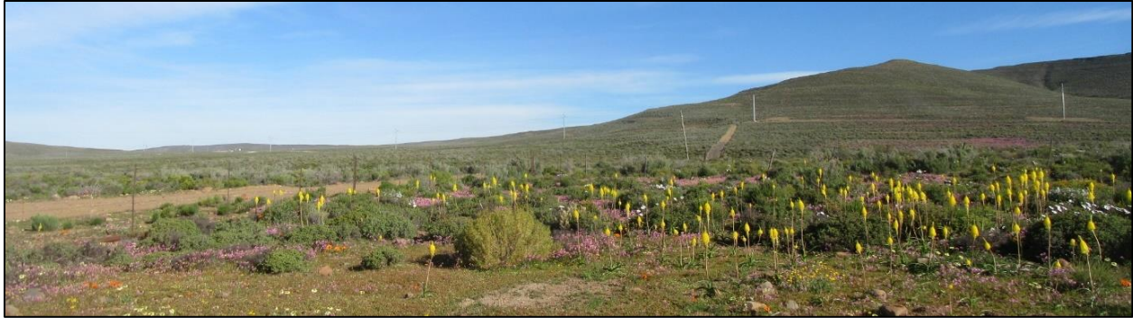
Photograph 3.12: Newly constructed line from the Roggeveld WEF to Eskom Komsberg substation, seen from access road to Bon Espirange
