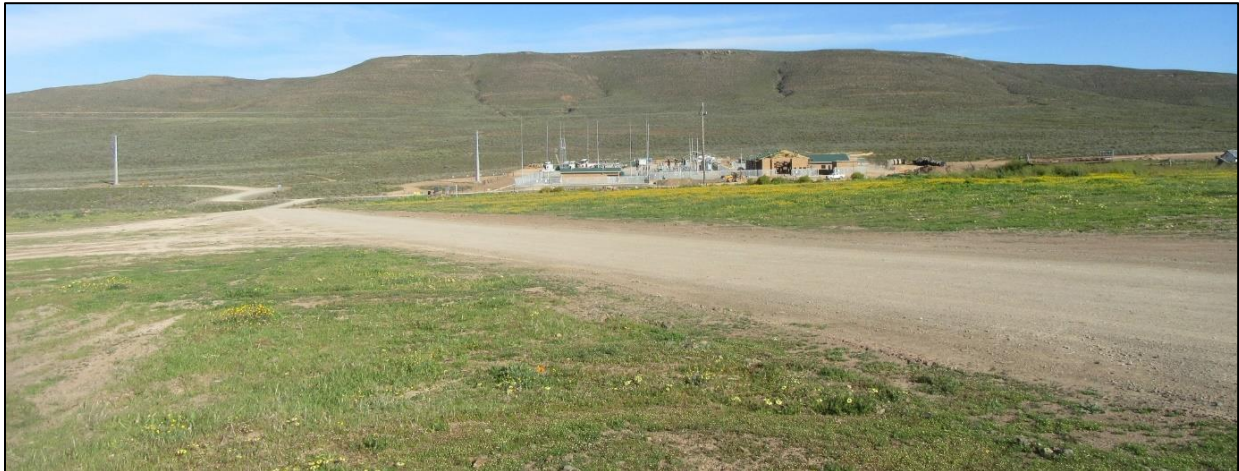
Photograph 3.10: Roggeveld WEF substation on Bon Espirange viewed from near the farmstead located to the north-west
