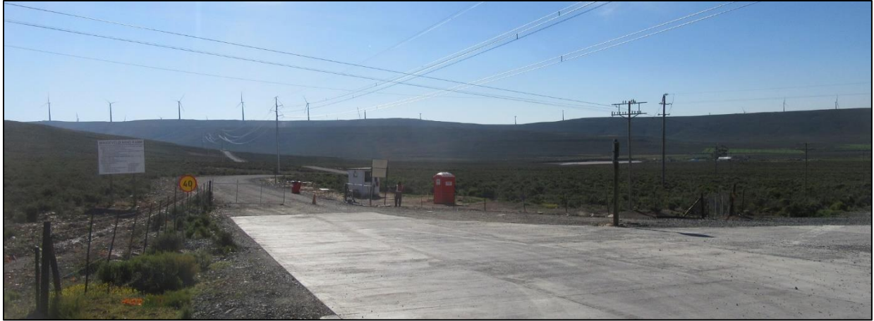
Photograph 3.9: Entrance to Roggeveld WEF from the R354 on Swartland
