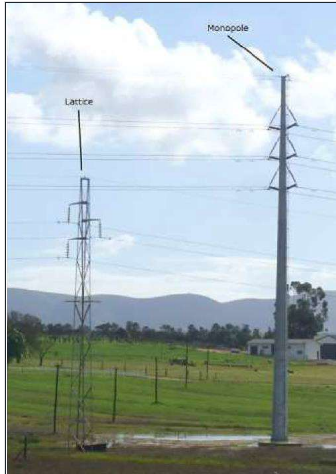
Figure 2-3 - Lattice Powerline Tower and Steel Monopile Structure
