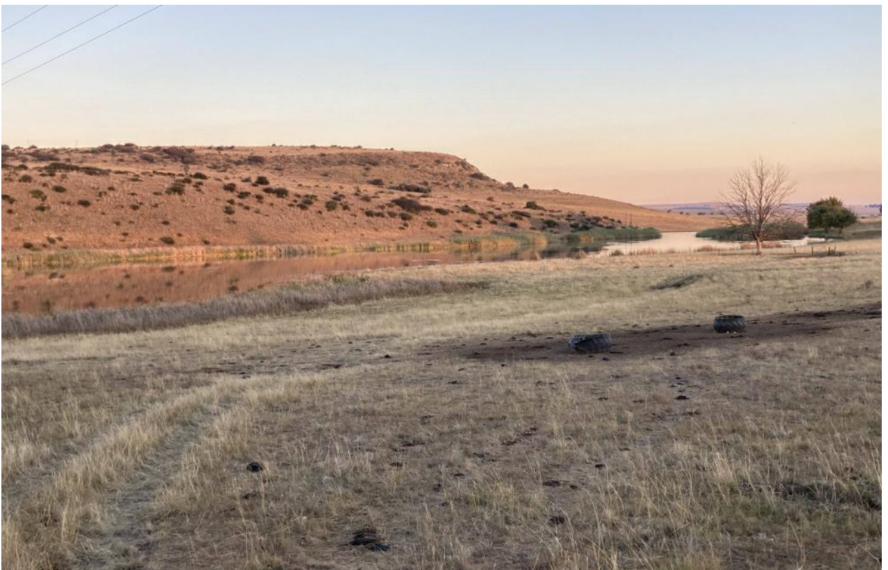
Figure 2: An example of an earth dam in the broader area
