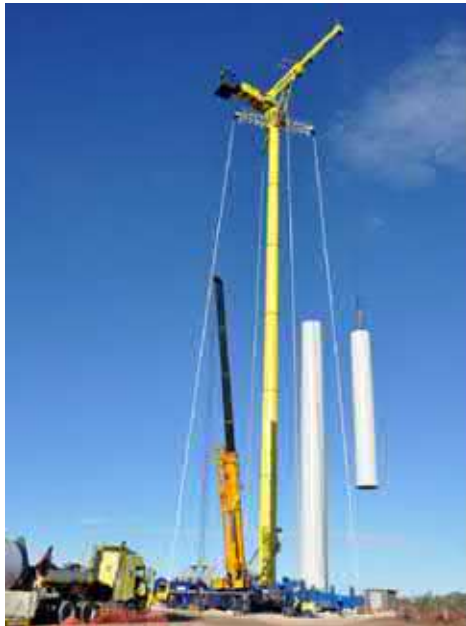
Figure 4-6: Cranes at work
