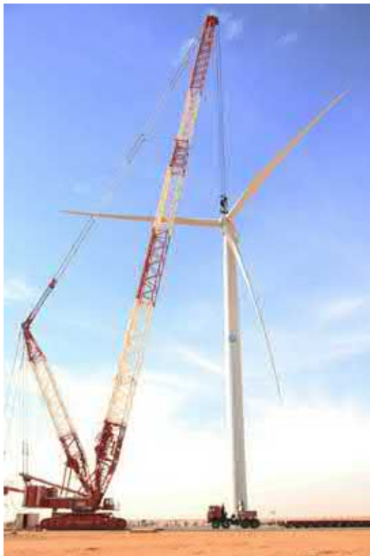
Figure 4-5: Crawler Crane used to assemble turbine (Liebherr, 2017)
