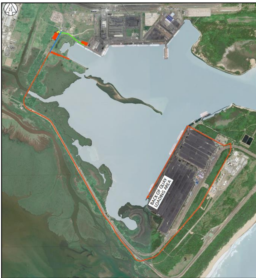
Figure 3-10: Existing access road to the proposed load-out berth
