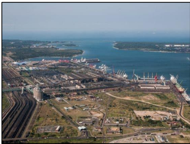
Figure 0-1: Overview of the Port of Richards Bay
