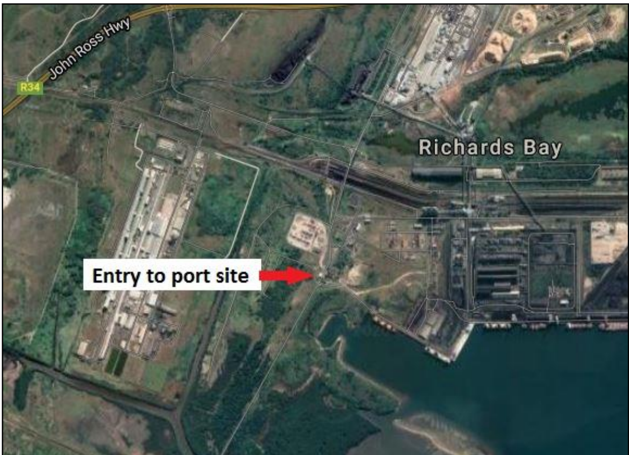
Figure 2-10: Google map showing existing access roads system to the Port of Richards Bay.
