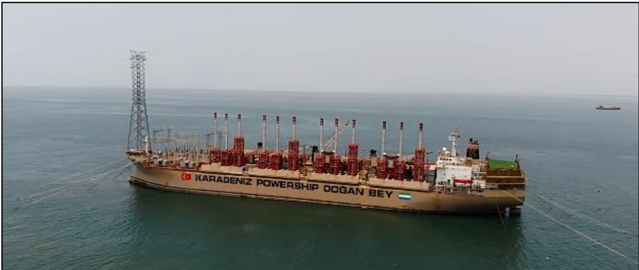
Figure 3-2: Powership mooring system.
