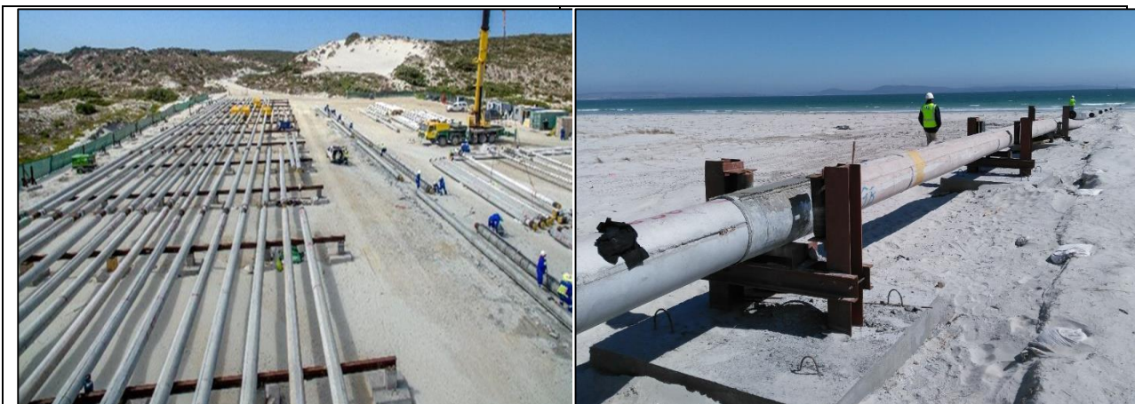
Figure 2-7: Typical Stringing Yard
