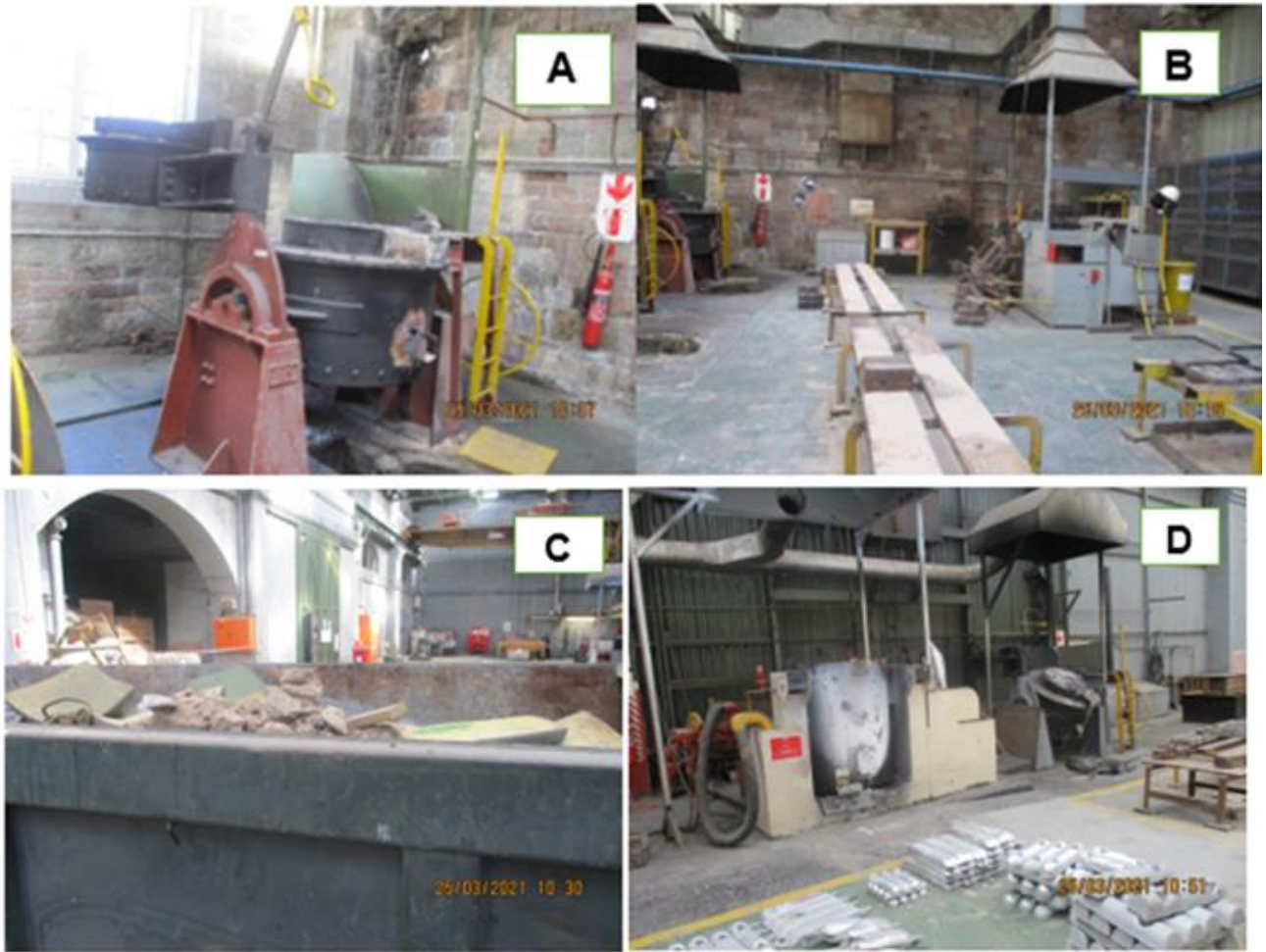
Figure 4: Images of the Armscor Dockyard foundry
