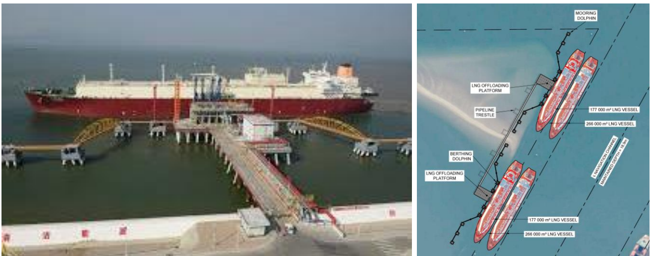
Figure 3: Left: Typical multiple piled concrete and steel quay; Right: Schematic design of the LNG Terminal capable of accommodating two LNG FSUs and/or vessels at the same time.
