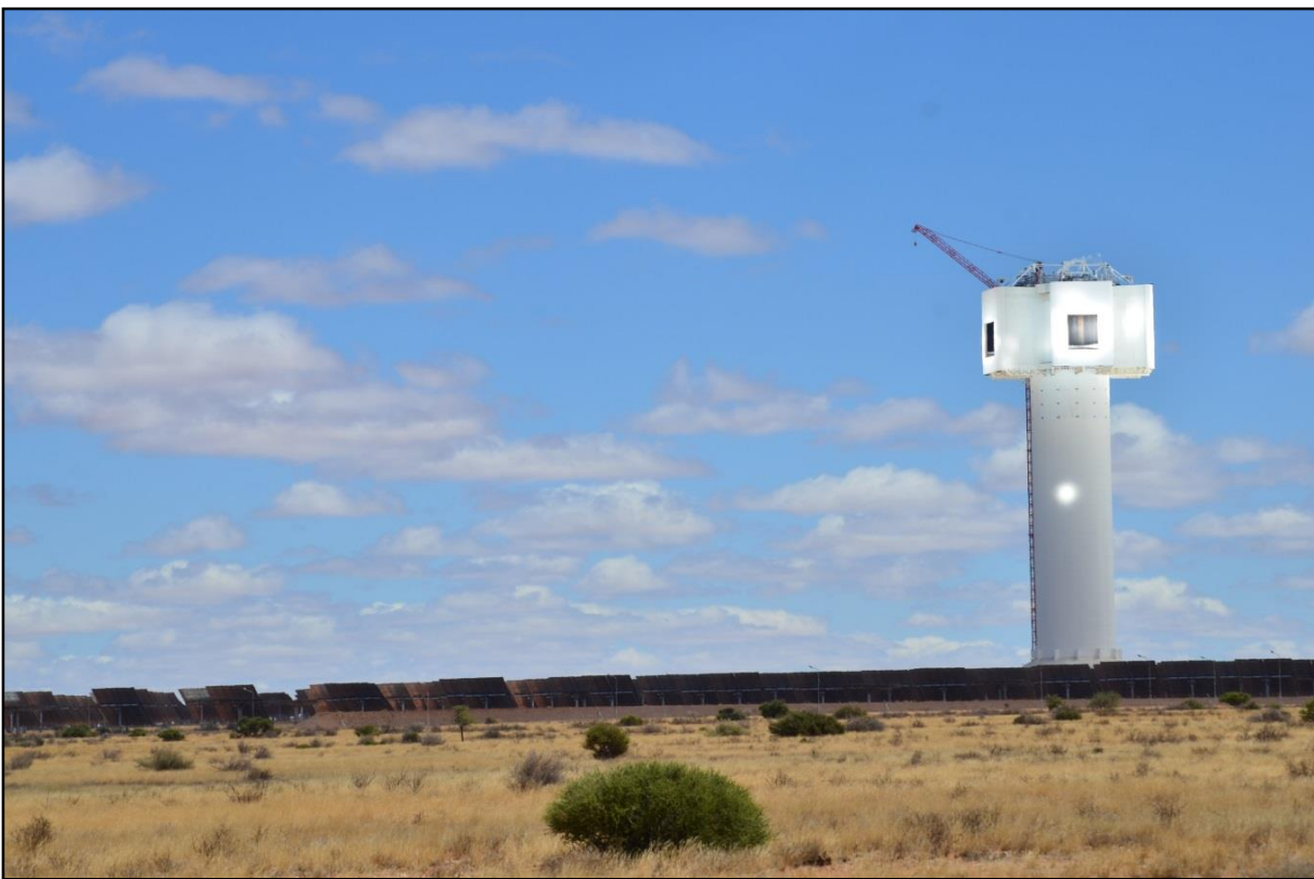
Figure 6-7: Kwi Solar One 50 MW CSP Tower facility currently under construction by Abengoa Solar near Upington, Northern Cape
