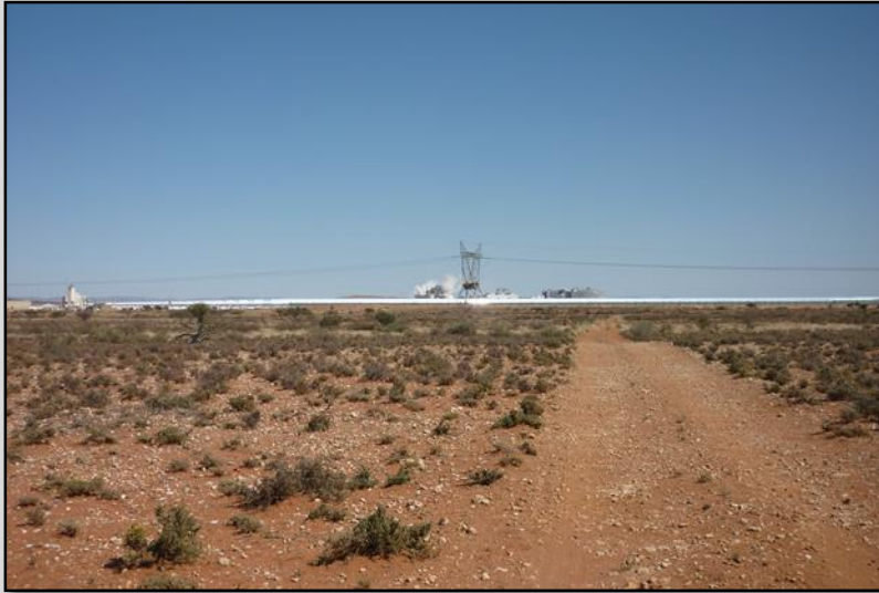
View of the project site from the eastern side.
