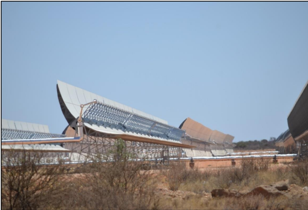
Figure 6-10: The Bokpoort I 75 MW CSP Trough Solar Development currently being commissioned near Groblershoop, Northern Cape
