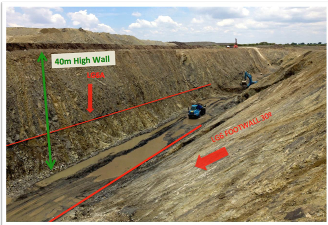
Figure 2-3: A view of the opencast pit and chromitite seams at nearby BCR mine
