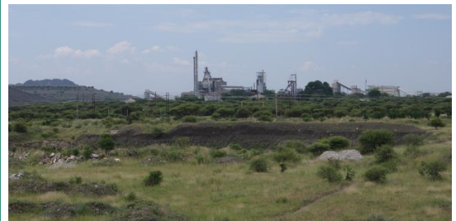
The existing Union mine constitutes the most prominent human element within the study area
