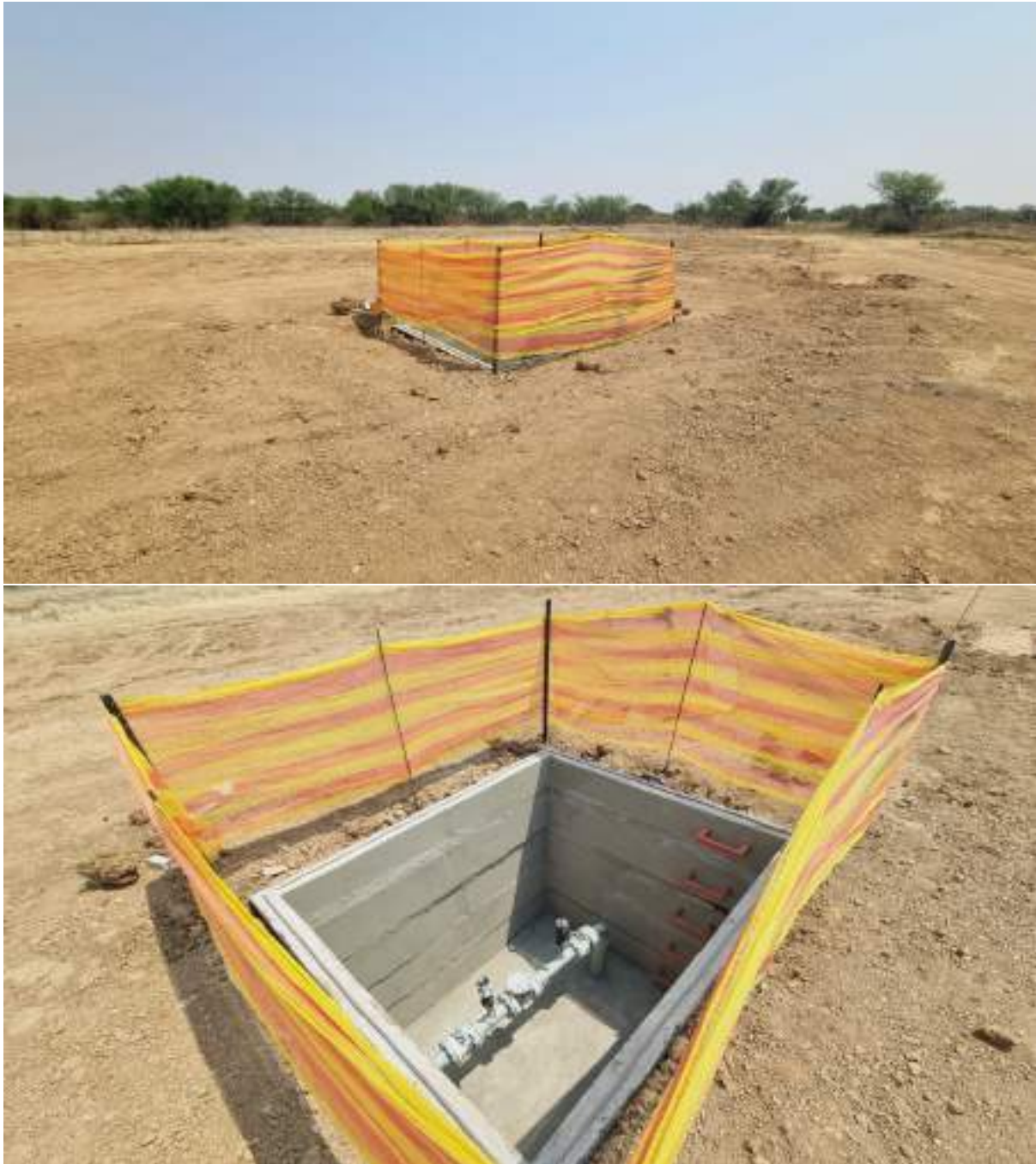
Figure 9: Typical example of a pre-cast well chamber.
