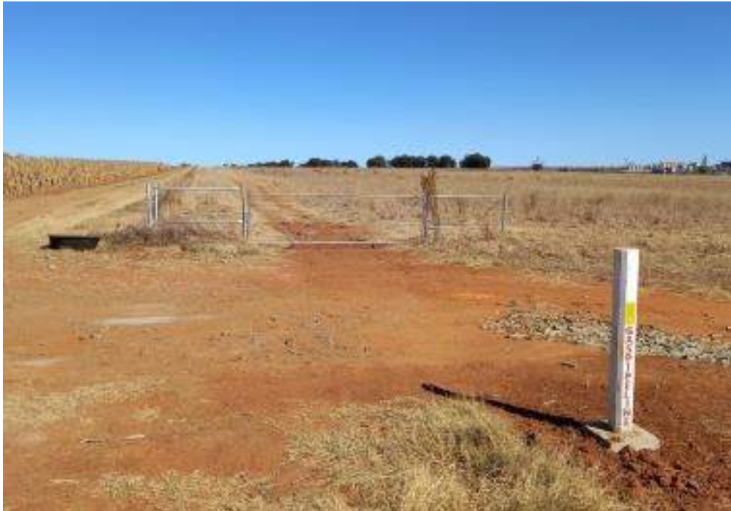
Figure 8: Typical pipeline servitude and pipe marker.
