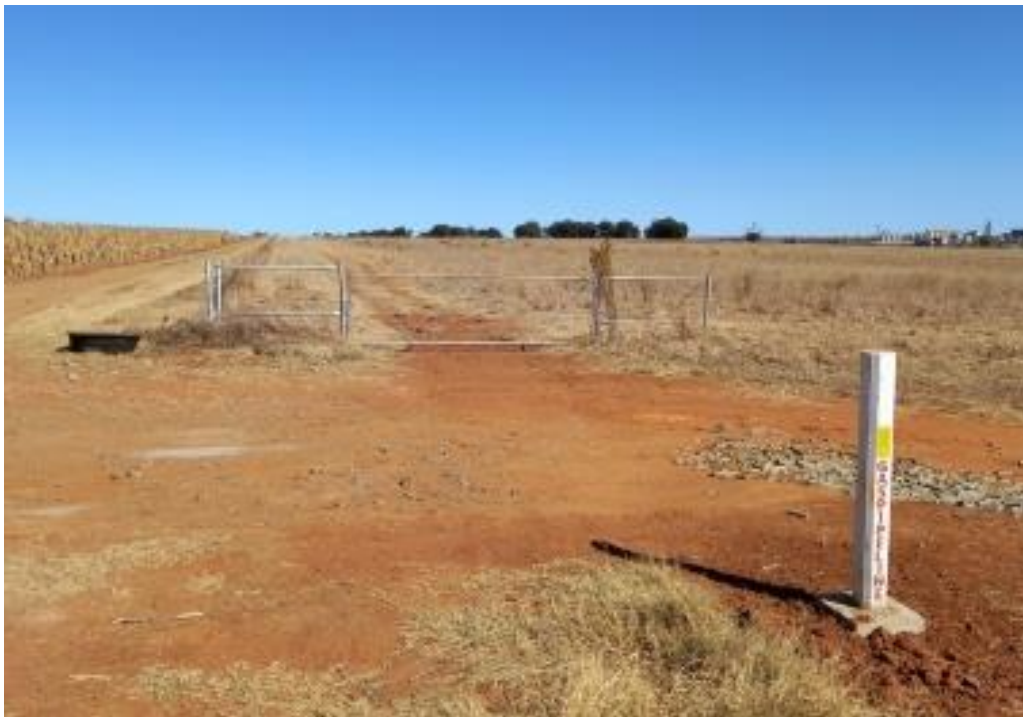
Figure 7: Typical pipeline servitude and pipe marker.
