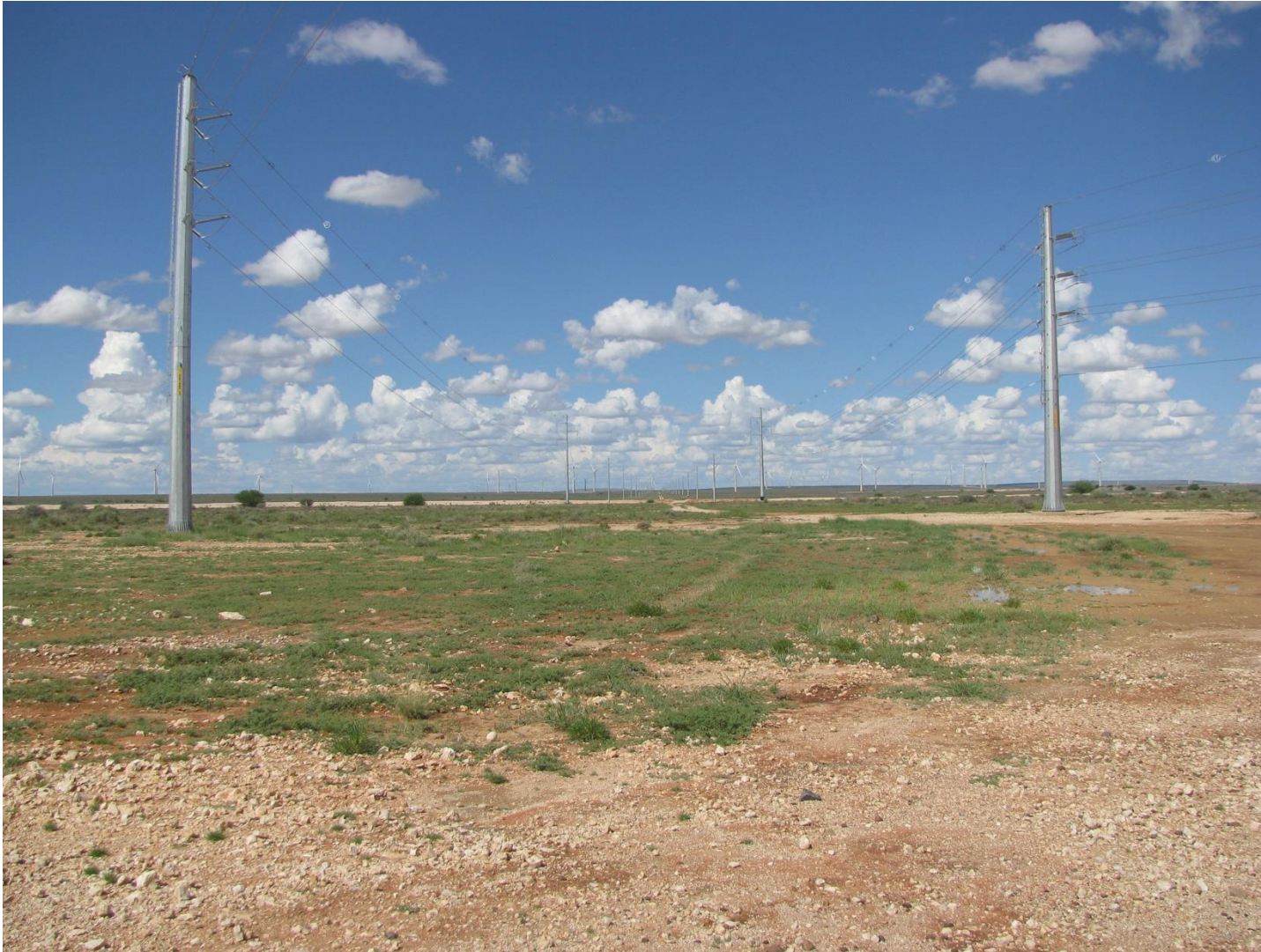
Figure 8-1 Some of the identified impacts within the project area: existing powerlines and fencing
