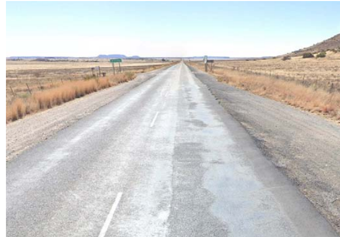
Photo 2: Northbound view along the R389 towards Kranskop Road
