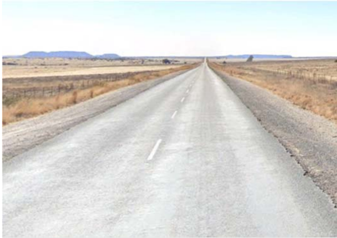
Photo 5: View to the north along R389 from Kranskop Road
