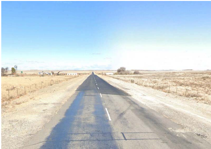
Photo 3: Southbound view along the R389
