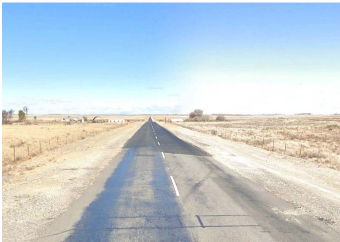
Photo 3: Southbound view along the R389
