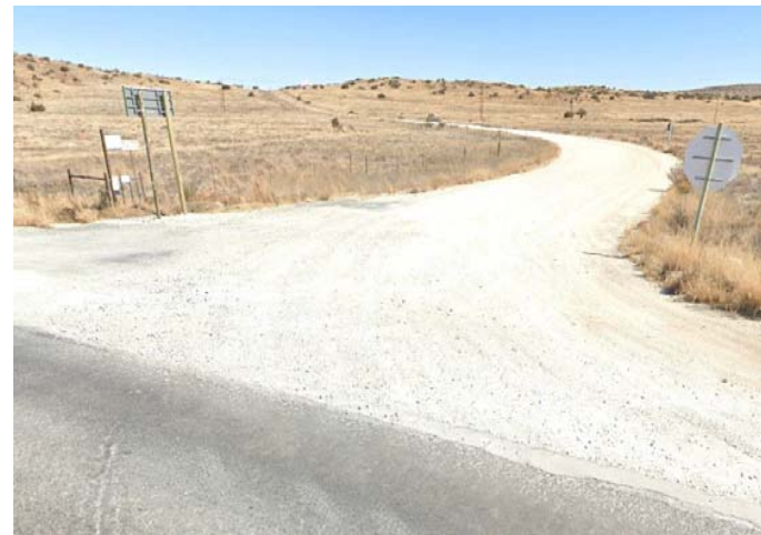
Photo 4: Westbound view Kranskop Road
