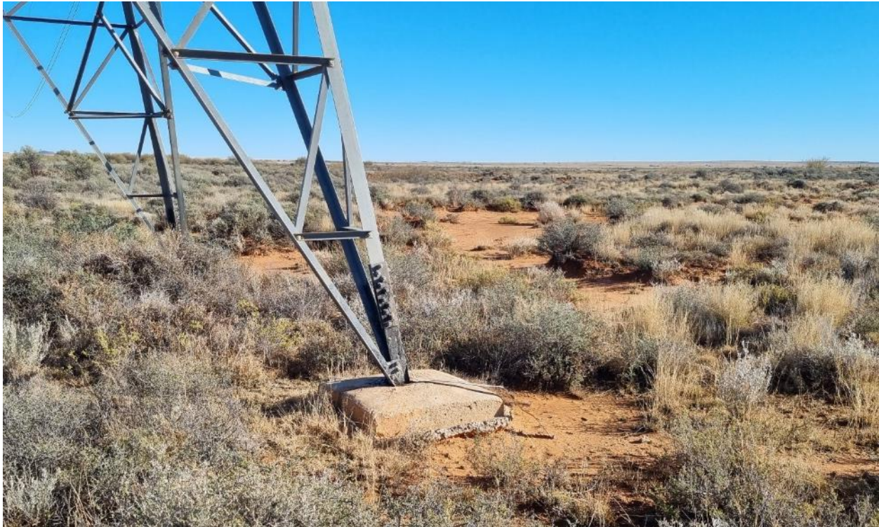
Figure 10-1: Concrete platform used to stabilise the electrical pylons
