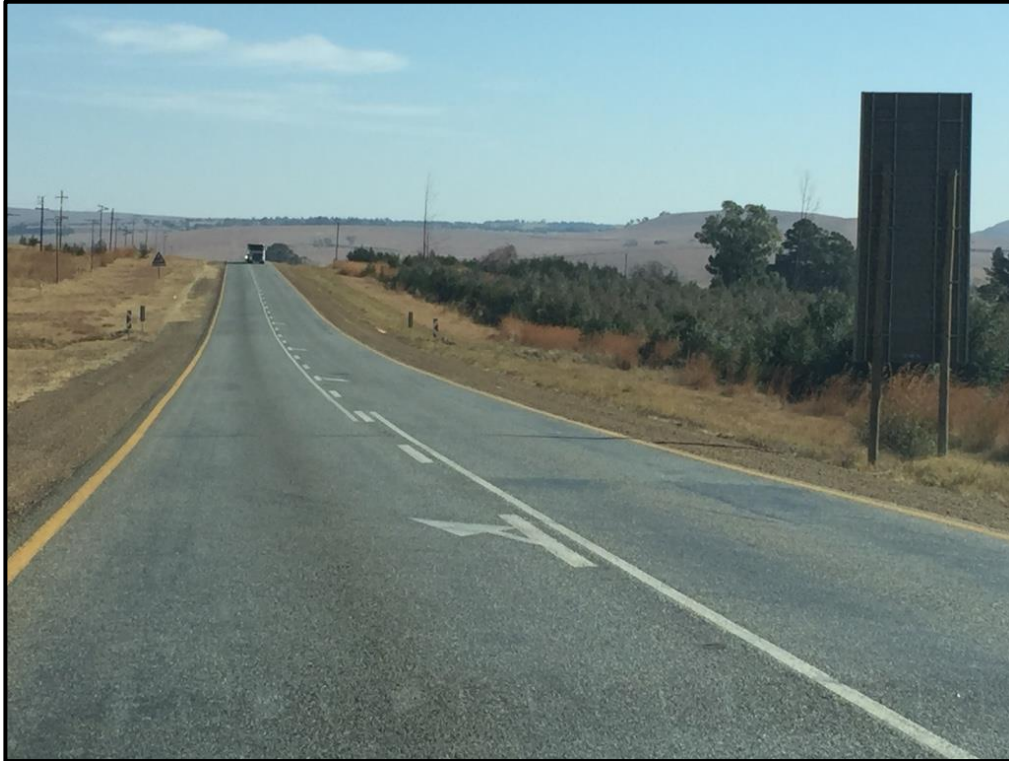
Photo 1: Section A at KM60,0 looking west along N2 Route
