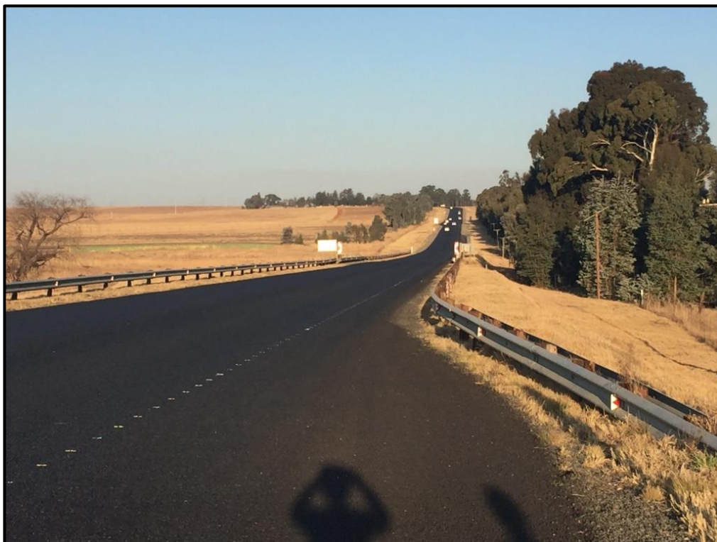
Photo 14: End of Section A at KM87,4. Looking SE back along the study area route
