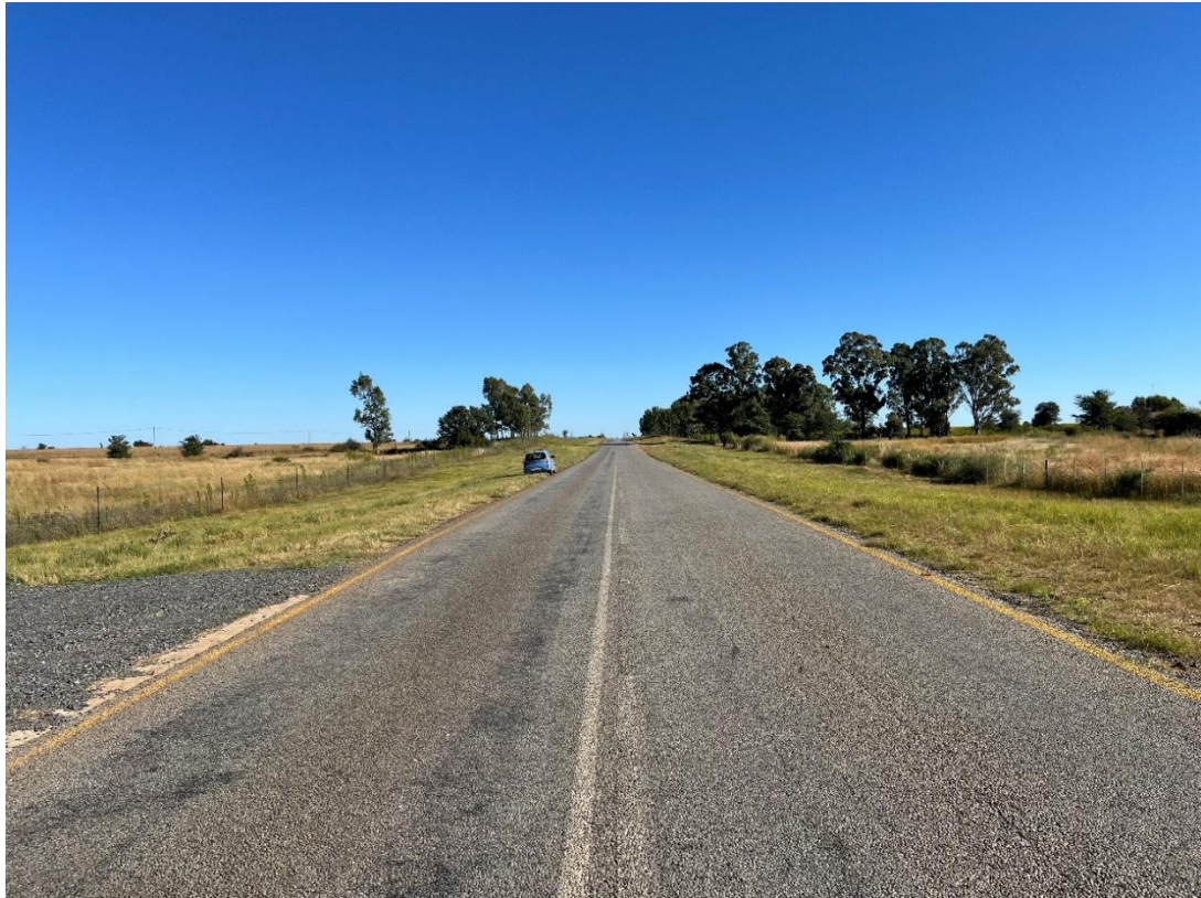
Figure 7:13 Existing Road R50505 @ Km 11.49 – North Approaching (Access 2)
