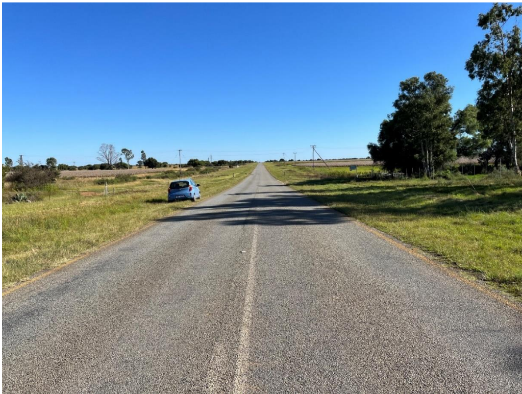
Figure 7:10 Existing Road R50505 @ Km 12.99 – North Approaching (Access 1)
