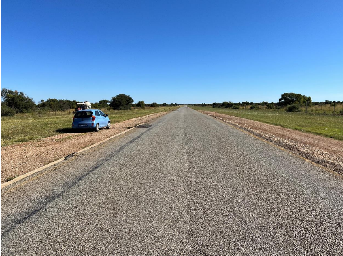
Figure 7:7 Existing Road R50505 @ Km 14.79 – North Approaching (Access 3)
