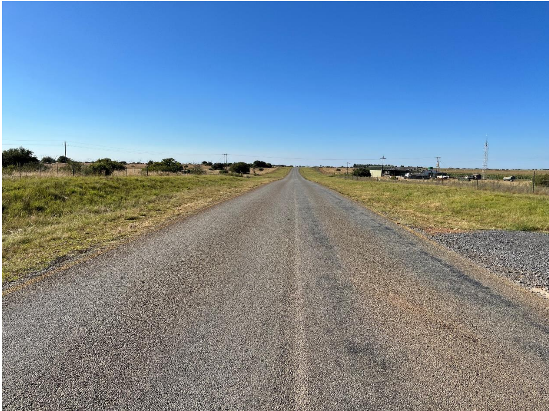
Figure 7:12 Existing Road R50505 @ Km 11.49 – South Approaching (Access 2)
