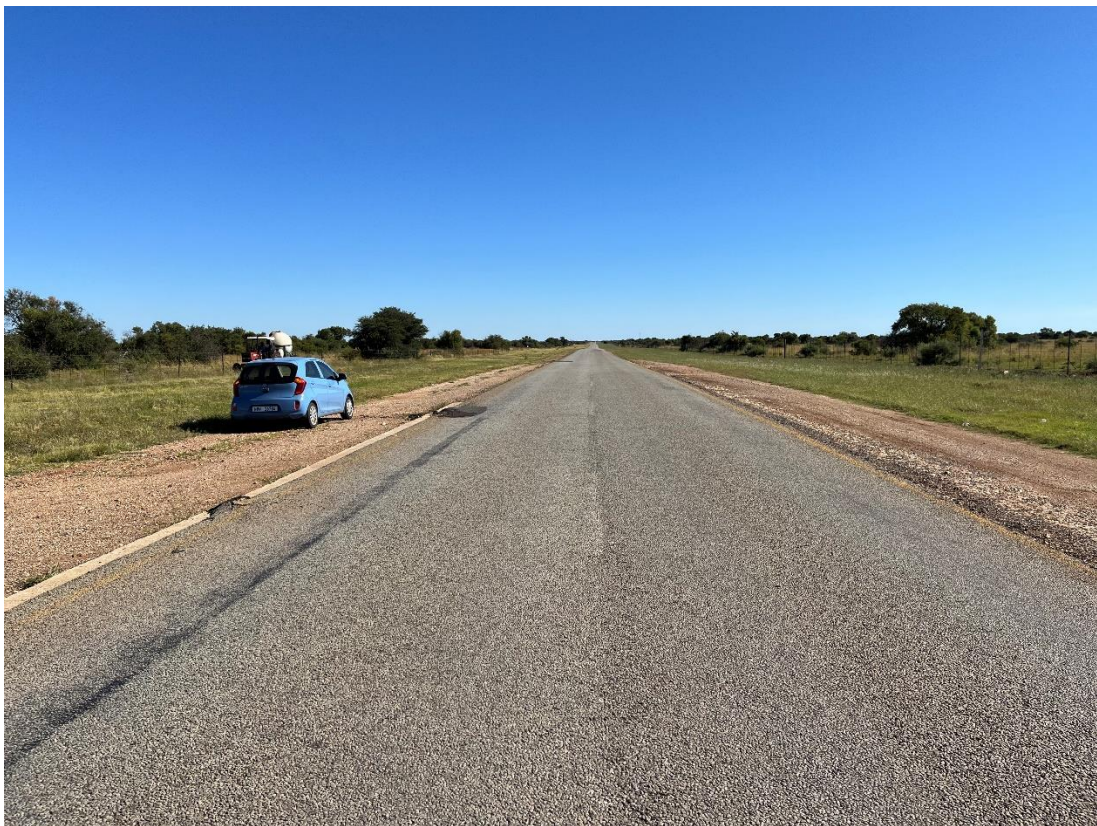
Figure 7:7 Existing Road R50505 @ Km 14.79 – North Approaching (Access 3)
