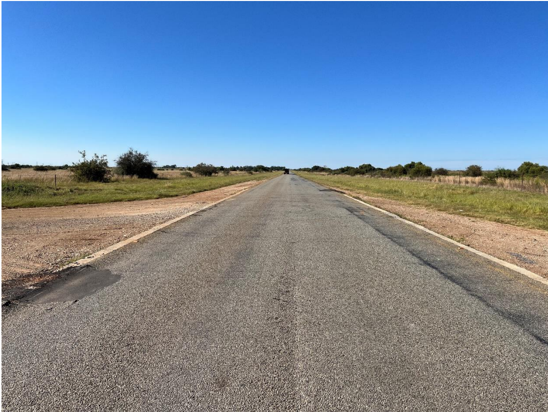
Figure 7:6 Existing Road R50505 @ Km 14.79 – South Approaching (Access 3)
