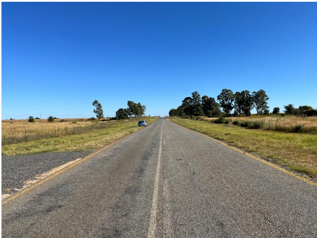
Figure 7:13 Existing Road R50505 @ Km 11.49 – North Approaching (Access 2)
