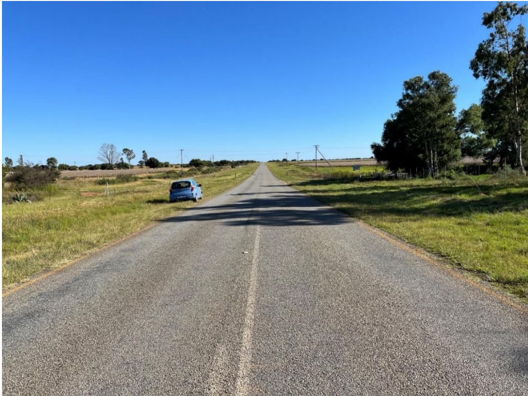
Figure 7:10 Existing Road R50505 @ Km 12.99 – North Approaching (Access 1)
