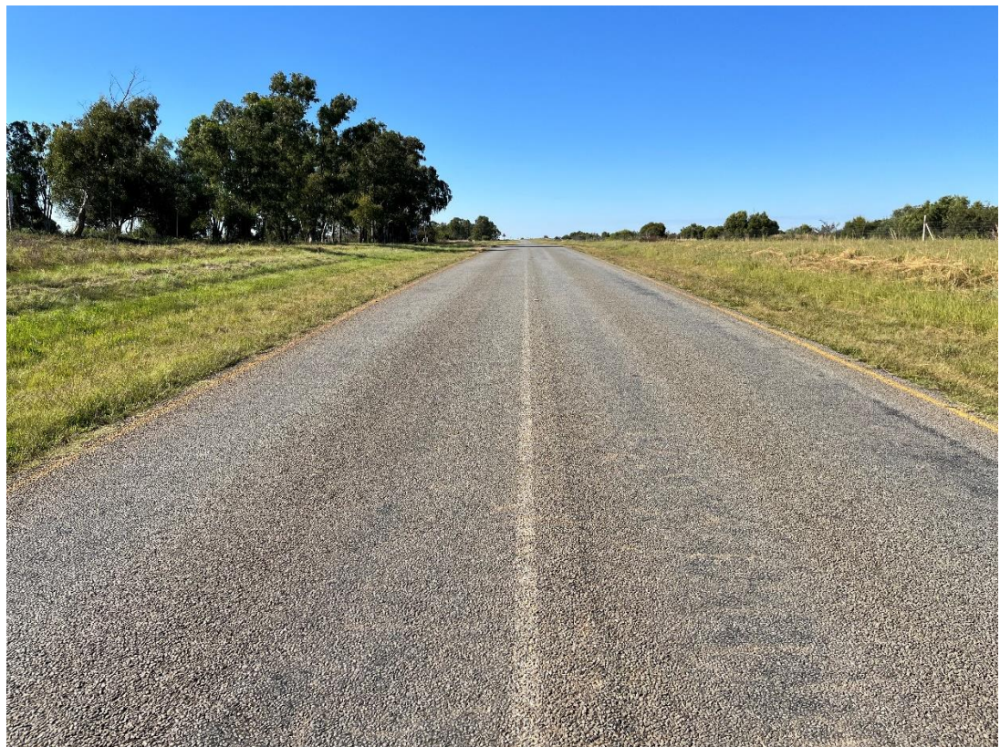
Figure 7:9 Existing Road R50505 @ Km 12.99 – South Approaching (Access 1)
