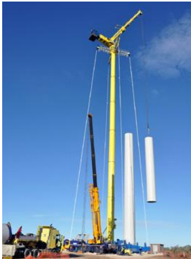
Figure 2-6: Example - Cranes at work
