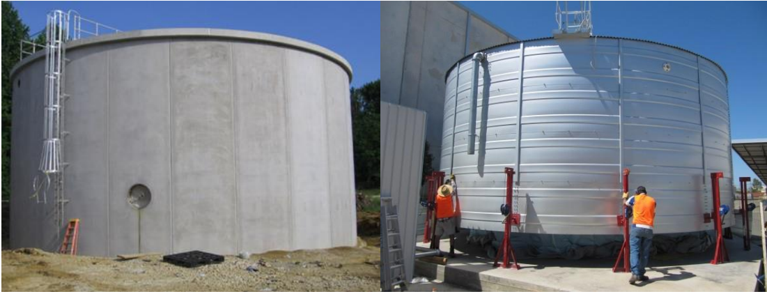
Figure 5 Typical water reservoir (left concrete, right steel tank ~ 6m).
