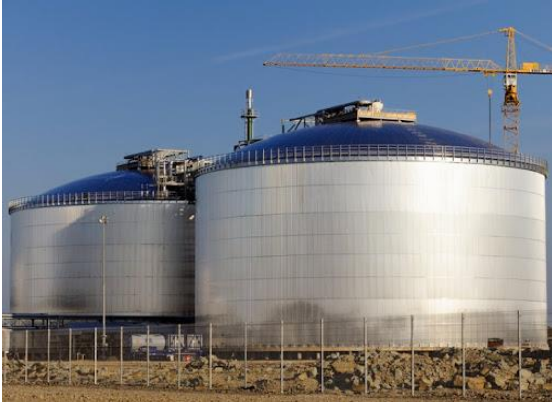
Figure 16: Cryogenic ammonia storage tanks
