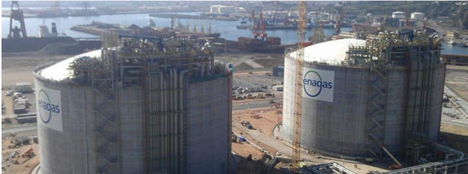
Figure 15: Liquid Ammonia Storage system (Energas example).
