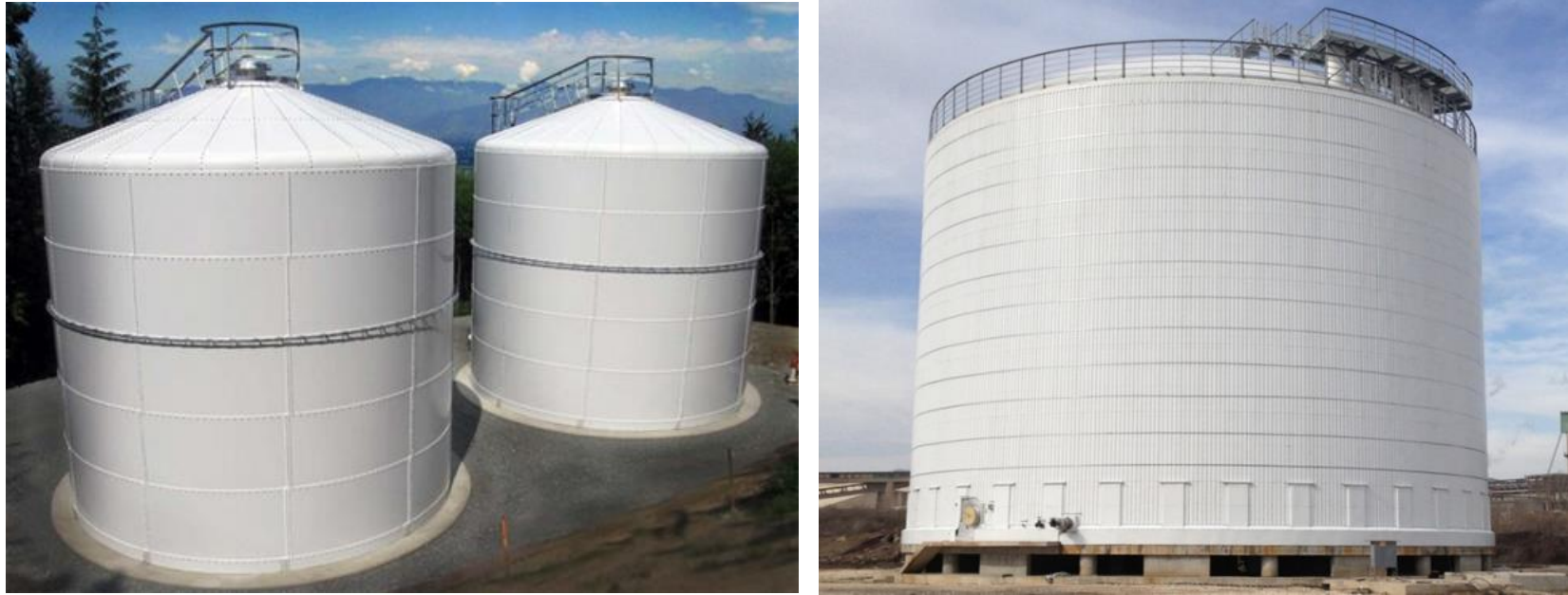
Figure 10 single-walled fixed storage tanks (left and double-walled fixed roof tank (right)
