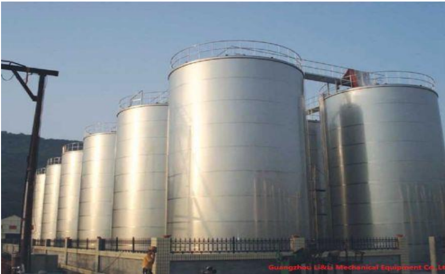
Figure 13: Stainless steel single-layered low-pressure tanks
