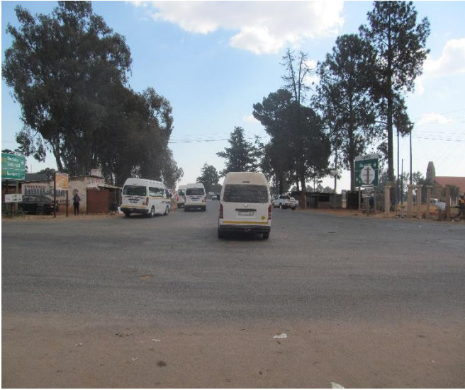
Photo 25: At km 38.9 towards the West
