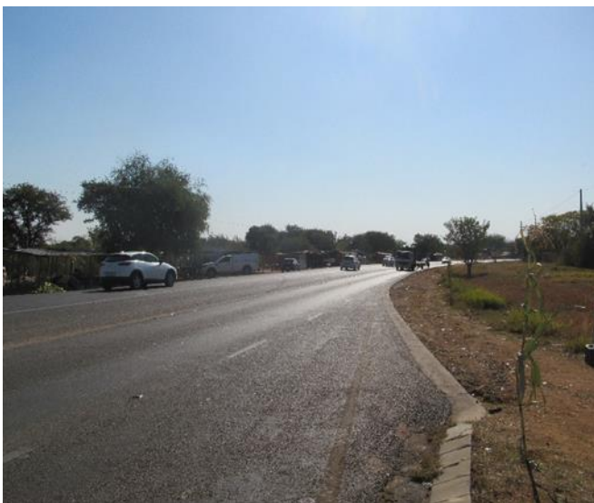
Photo 9: Towards the North at km 0
