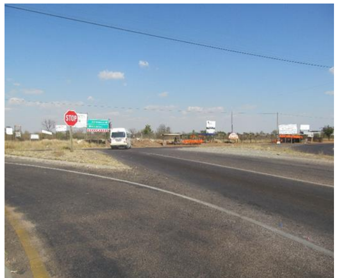
Photo 10: Towards the South at km 0
