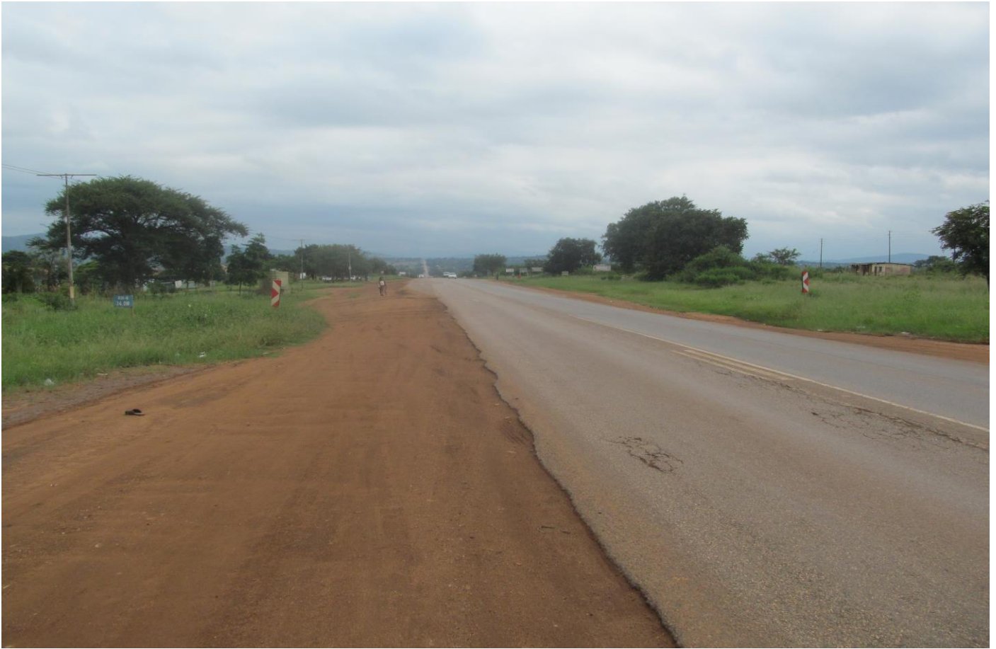
Photo 13: At km 14 towards the North East
