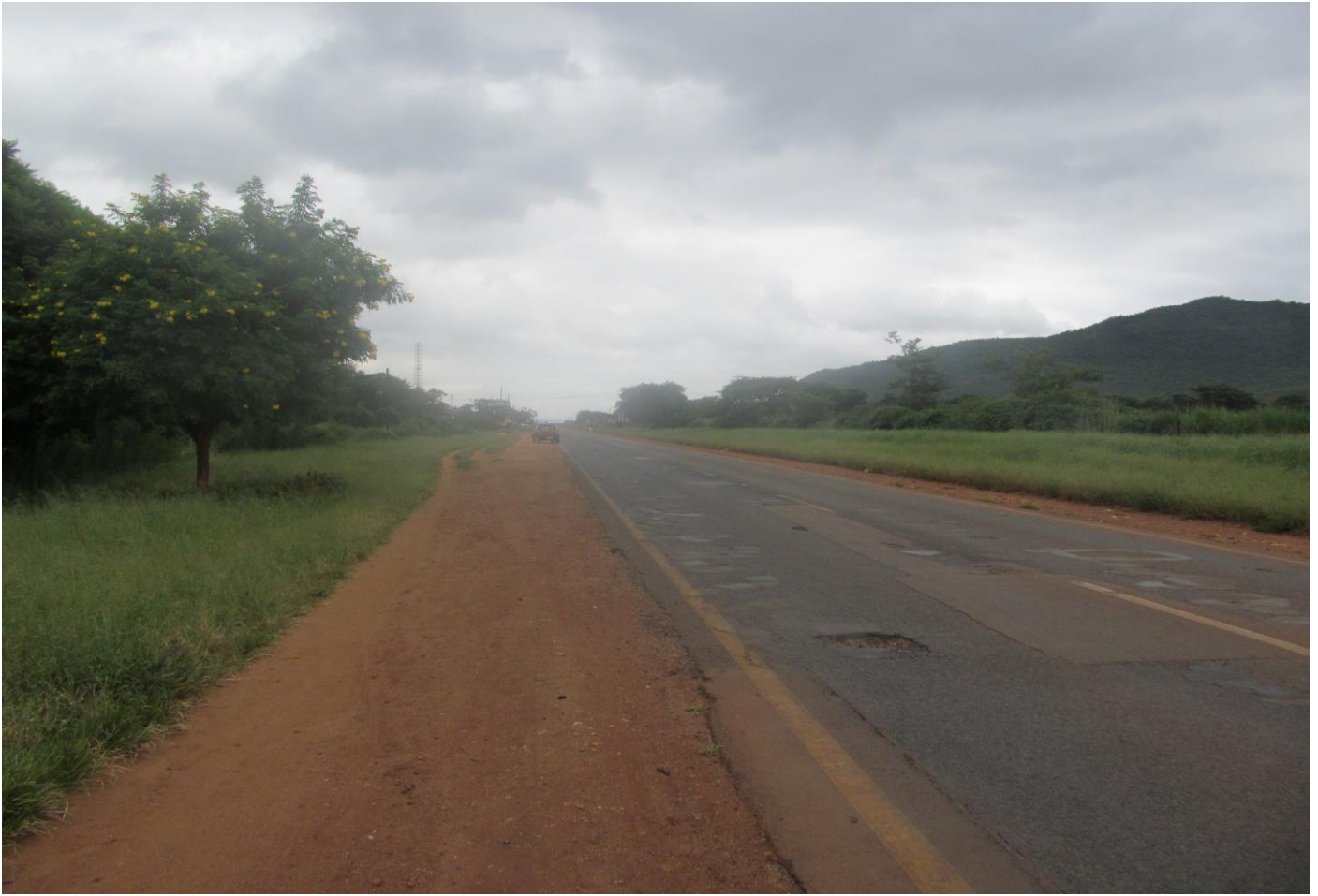
Photo 9: At km 4.7 to the North West
