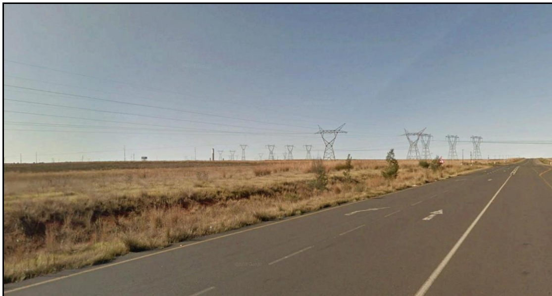
Figure 11: Power lines near the R542 arterial road.
