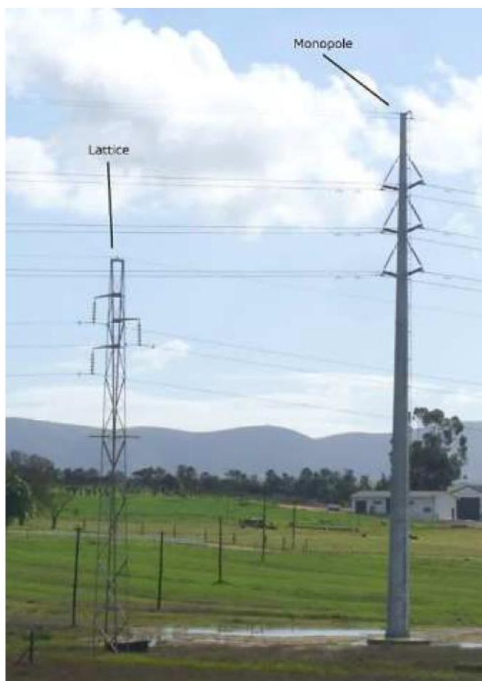
Figure 3-4: Conventional lattice powerline tower compared with a steel monopole structure
