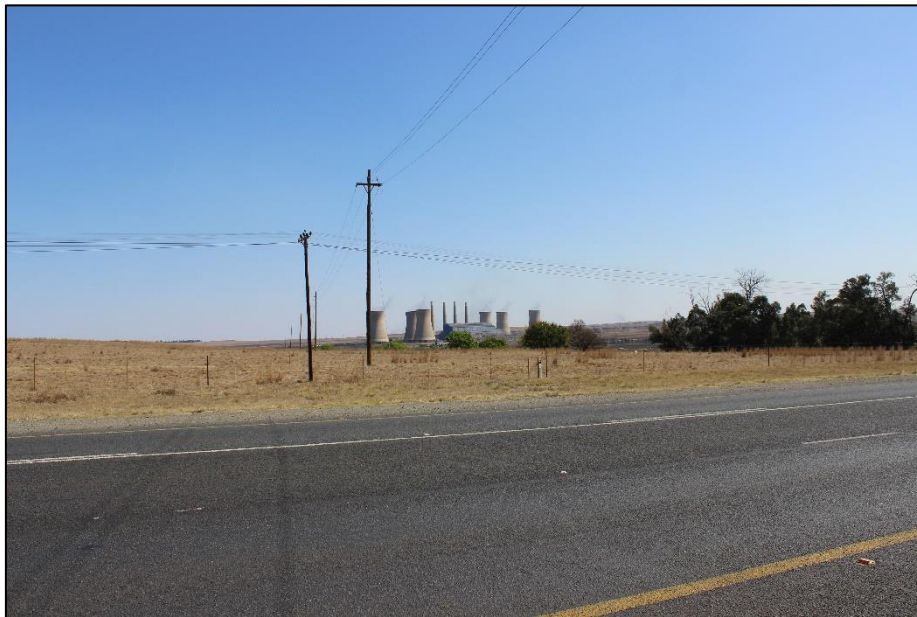
Figure 16: View of Camden Power Station to the west of the N2 national route.
