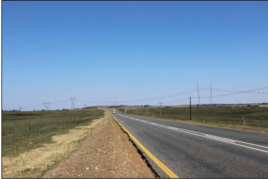
Figure 17: High voltage power lines feeding into Camden Power Station.
