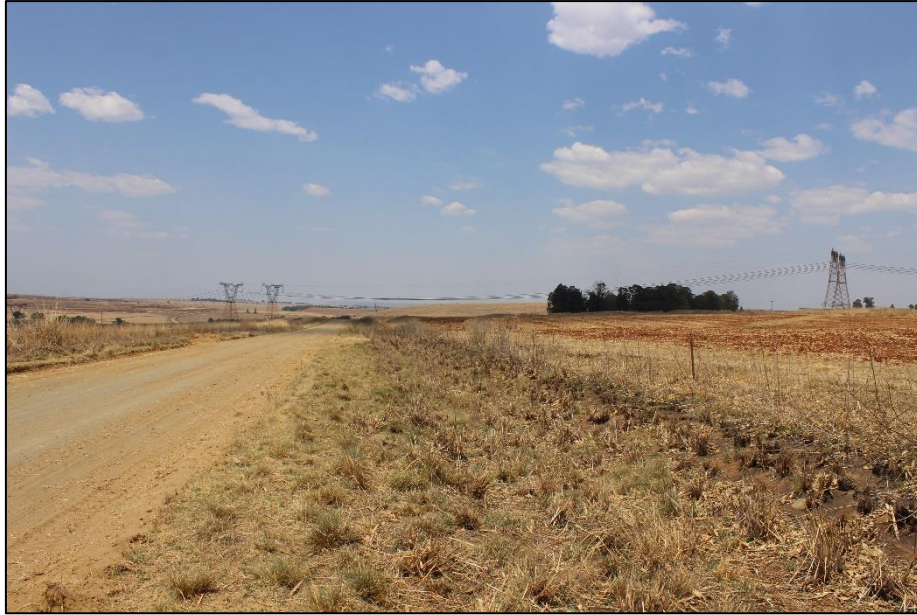
Figure 18: High voltage power lines feeding into Camden Power Station.
